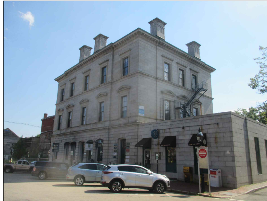
EXISTING NORTH EAST BUILDING CORNER
