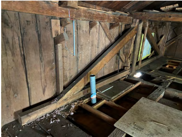
23-Modified framing to bridge over the removed post and wall at lower level
