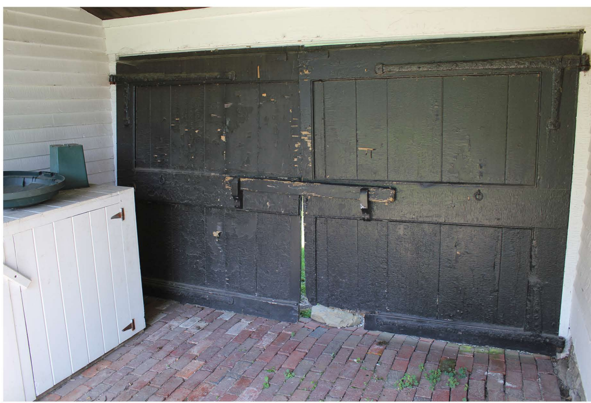
POSSIBLE HISTORIC DOOR WITH HISTORIC HINGES
