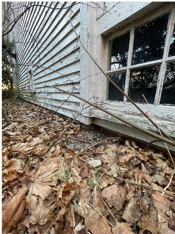
NEW WINDOW REPAIR
