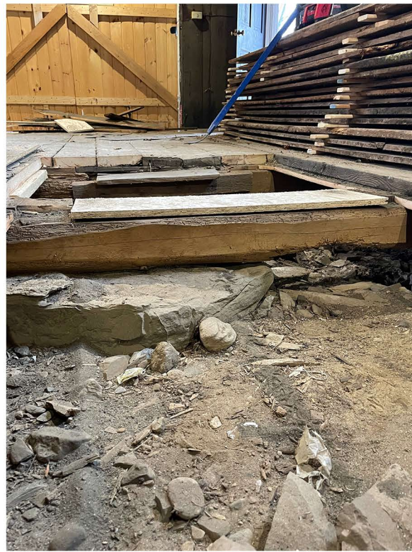
TYPICAL BEAMS IN DIRECT CONTACT WITH GROUND
