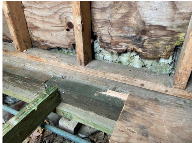
4-Connector inside face of brick cladding
