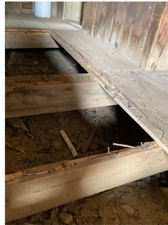
TYPICAL FLOOR FRAMING MADE UP OF REPURPOSED BEAMS
