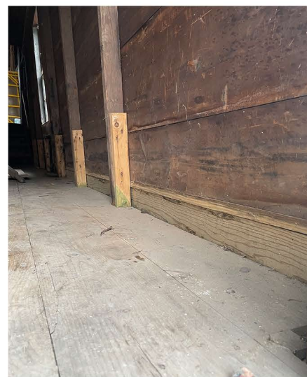
PRESSURE TREATED SILL REPAIR
