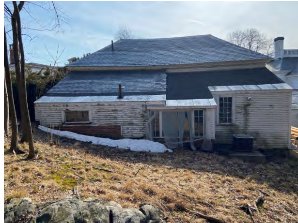
18-Carriage house northeast elevation
