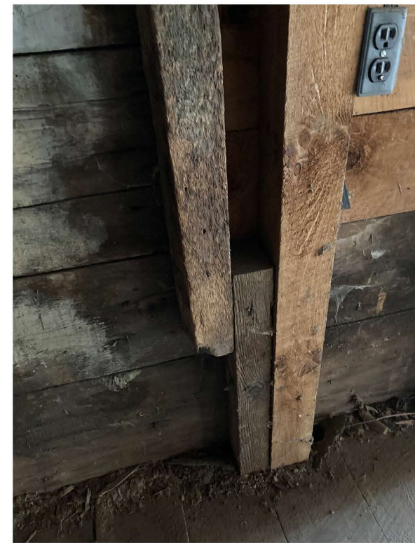
TYPICAL FRAMING AT FRONT WALL
