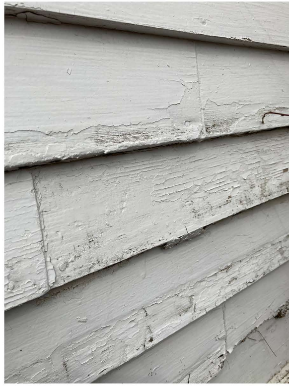
TYPICAL SIDING BUTT JOINT
