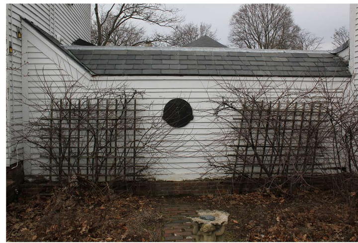
VIEW OF EXISTING SIDE ELEVATION
