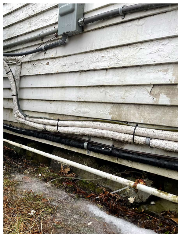
STONE RUBBLE FOUNDATION
