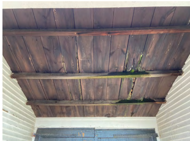
14-Connector roof sheathing and purlins
