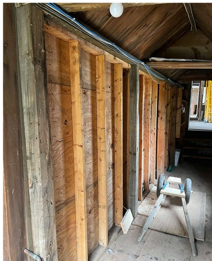
INTERIOR STUDS / PLYWOOD
