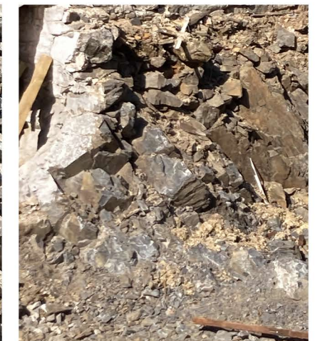
6. EXISTING FOUNDATION AT MANSION
