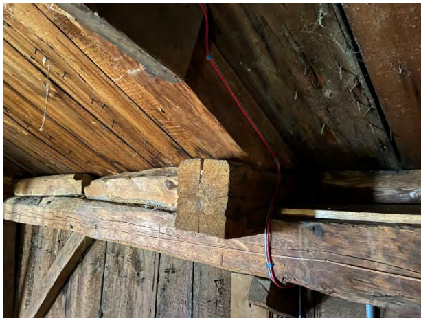
21-Cut bottom chord on line 7.5
