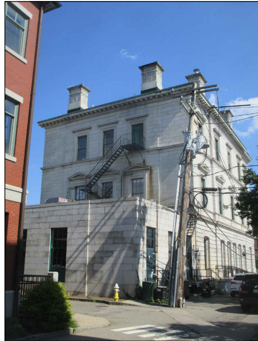
EXISTING NORTH WEST BUILDING CORNER
