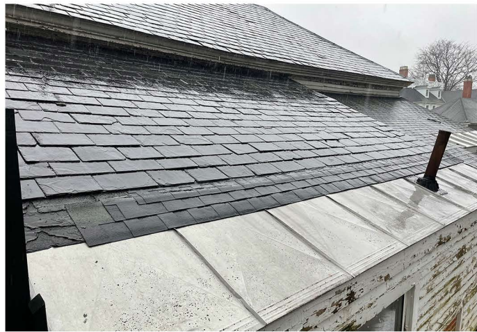
SLATE, ASPHALT AND, METAL ROOFING
