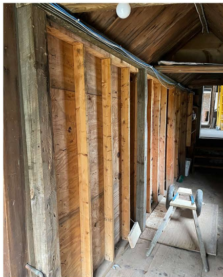
INTERIOR STUDS / PLYWOOD
