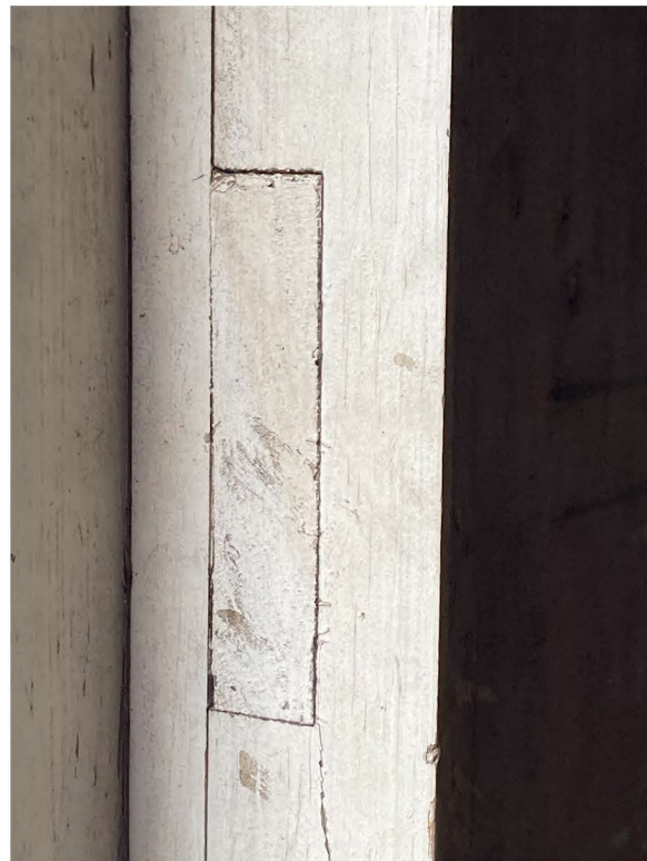
BARN DOOR MORTISE AND TENON
