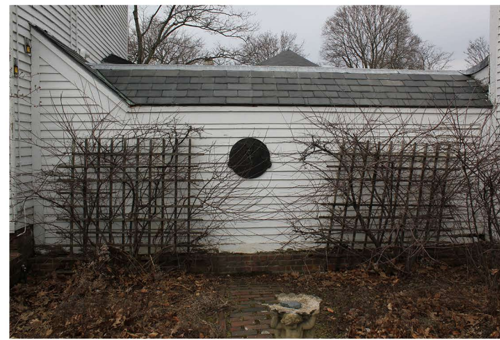
VIEW OF EXISTING SIDE ELEVATION
