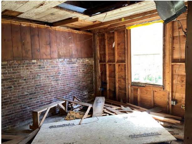
19-Brick foundation and front wall framing
