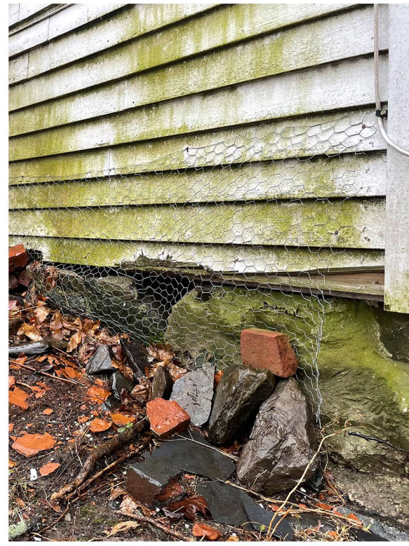
STONE RUBBLE FOUNDATION AND NEW SIDING REPAIR
