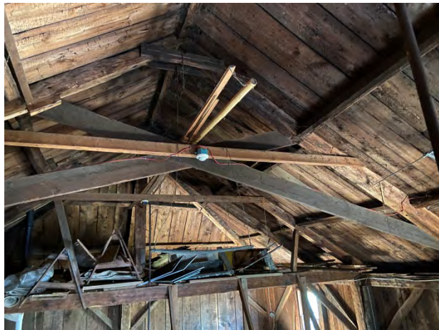
22-Modified roof framing at line 7.5
