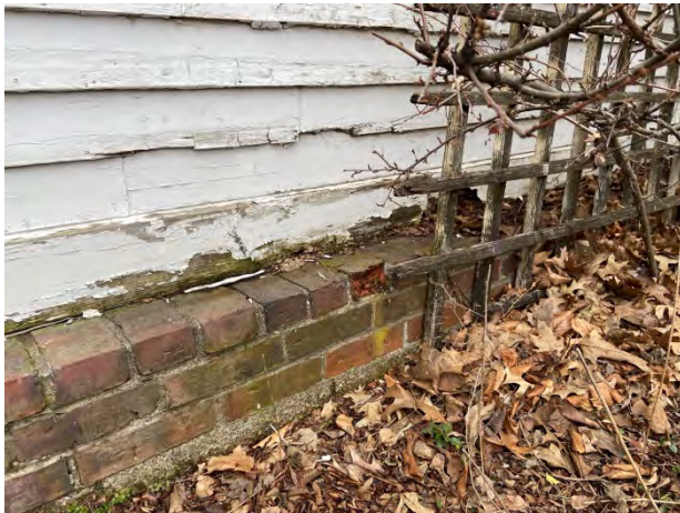
3-Connector brick cladding on south side
