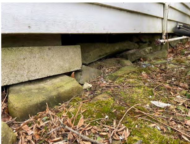
5-Connector foundation on north side
