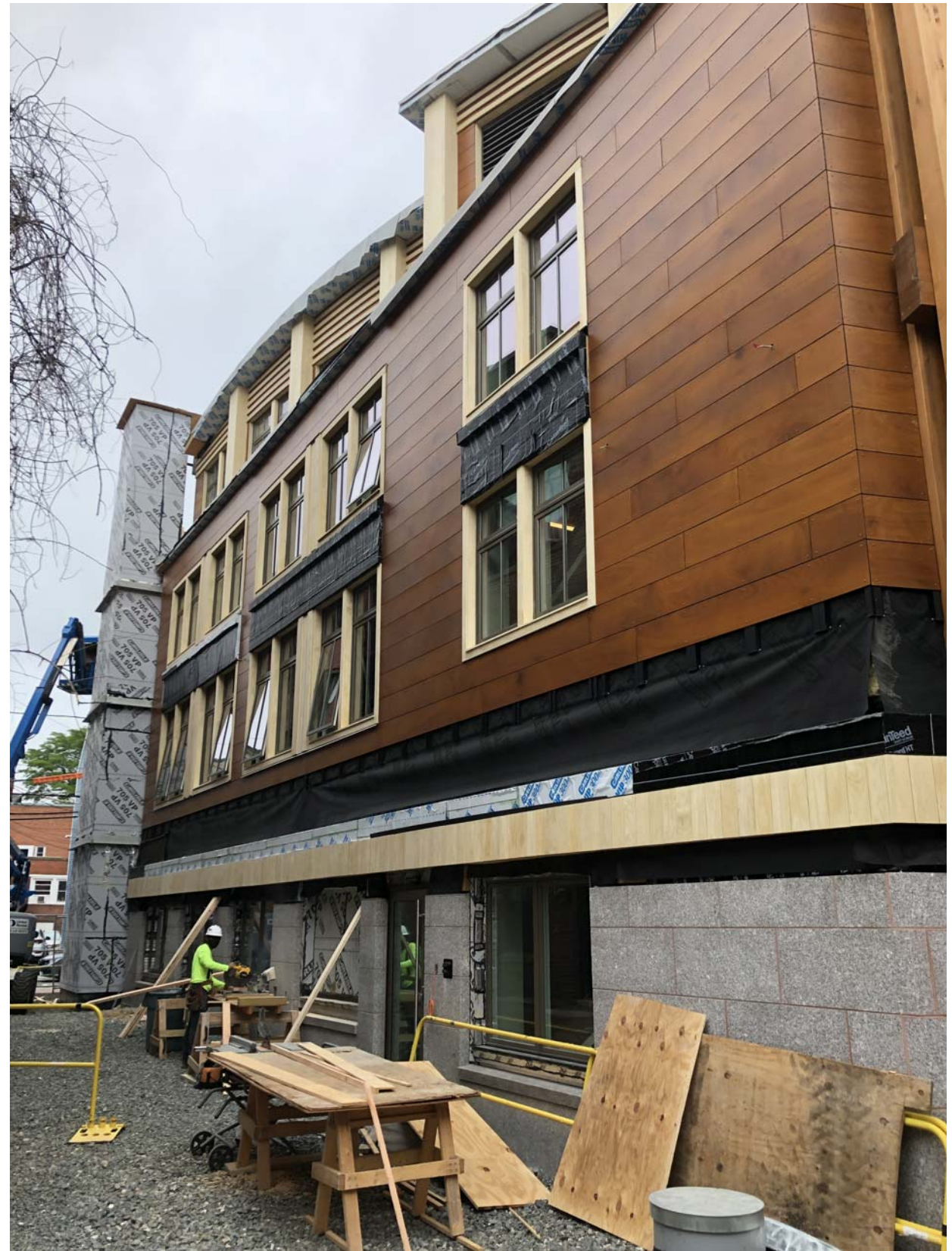
PHOTO OF INSTALLED WEST FACADE
