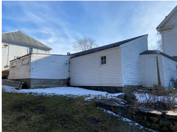
8-Barn north elevation
