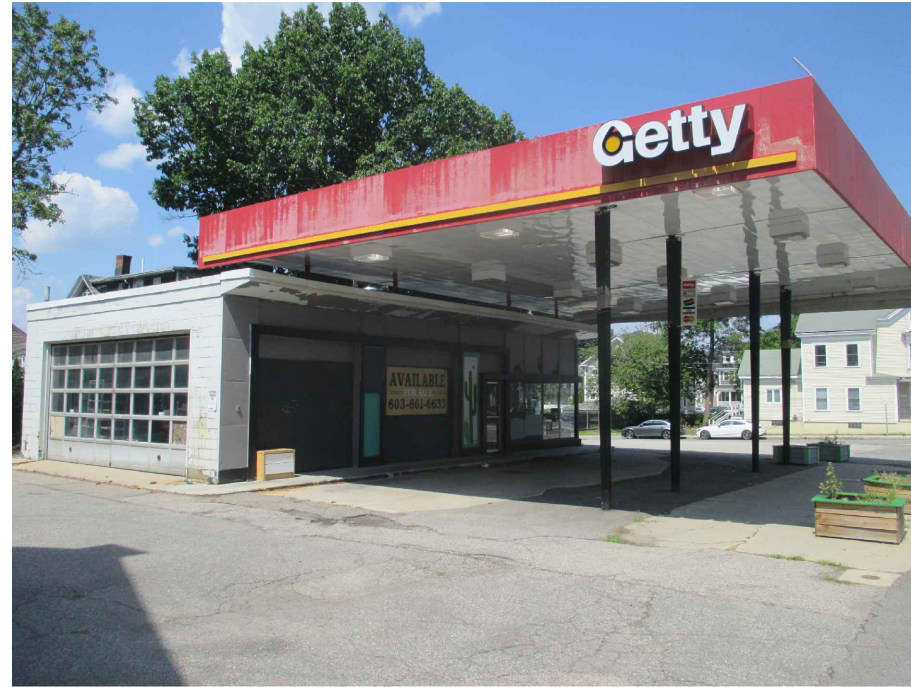
EXISTING VIEW FROM SOUTH WEST
