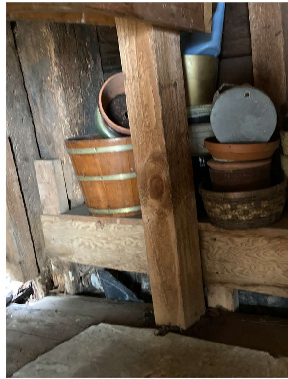
REPAIRS AT COMPROMISED STRUCTURE AT BASE
