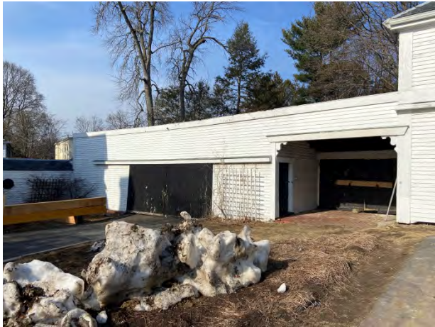
7-Barn southwest elevation
