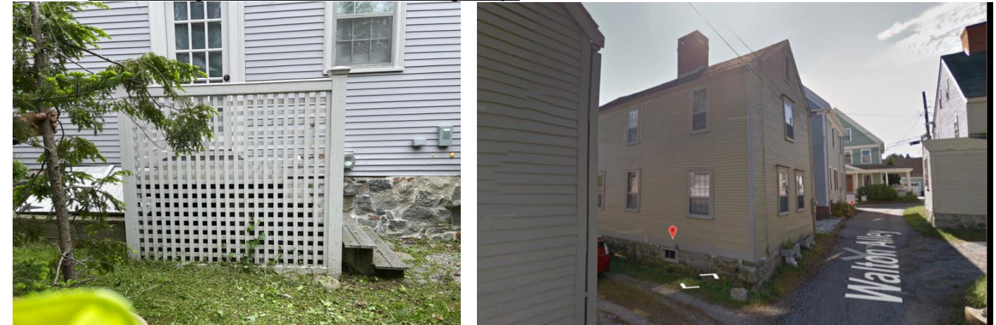
Rear Elevation and Streetscape View
