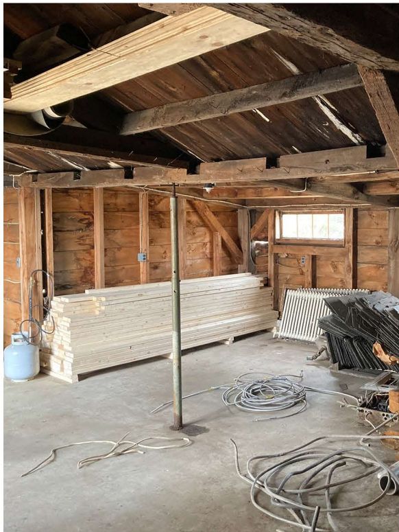
NEW FRAMING AT 1979 CARPORT
