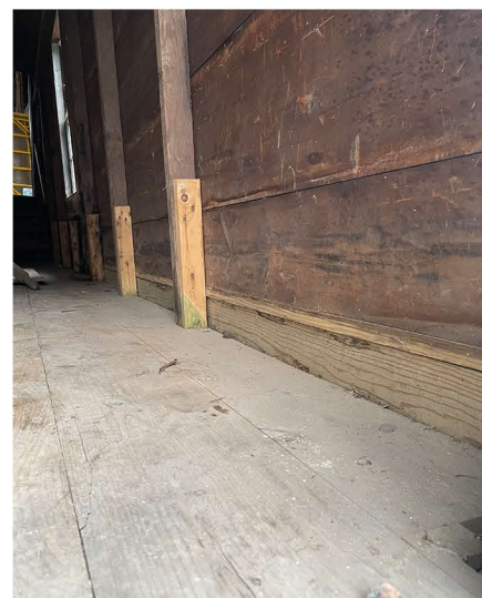
PRESSURE TREATED SILL REPAIR
