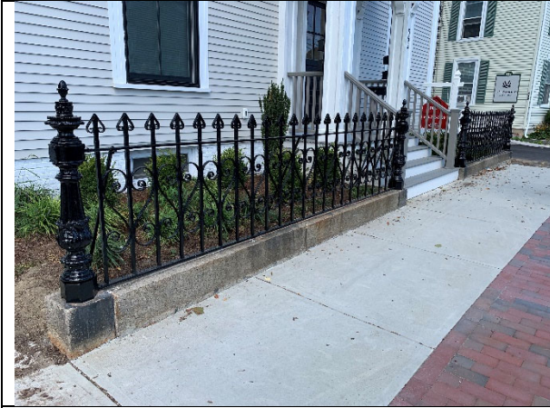
Wrought iron fence repaired
