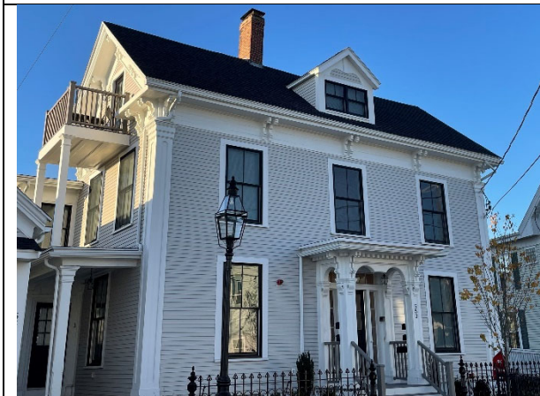
Completed dormer with added trim
