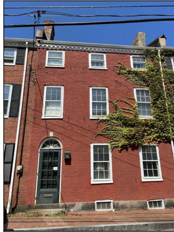
23.) 17 SHEAFE STREET: 24' - 4" (F)
