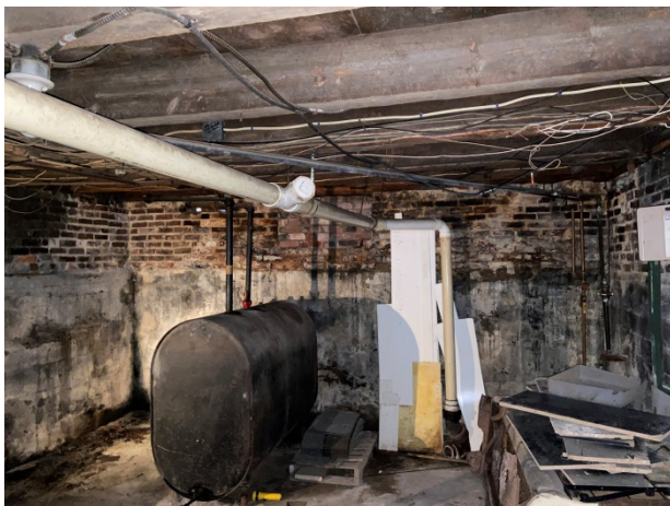
23-Basement looking north
