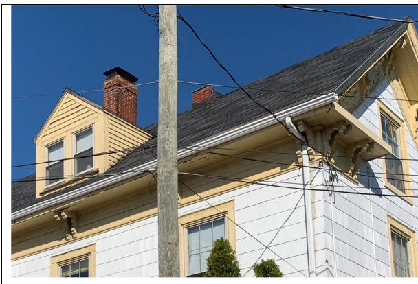
Original chimney, capped at ridge
