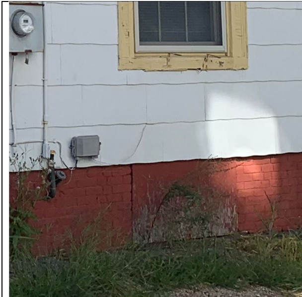
Original Basement window opening boarded up
