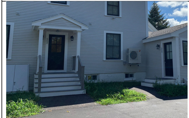
Bulkhead relocated, stair landing simplified
