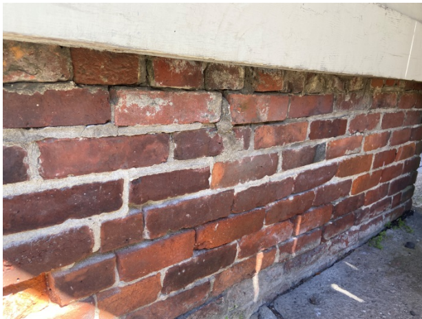
21-East side brick foundation wall
