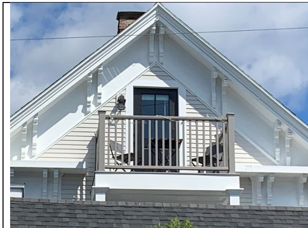
4-light door at Third Floor Deck
