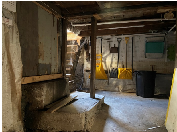
8-Basement looking south
