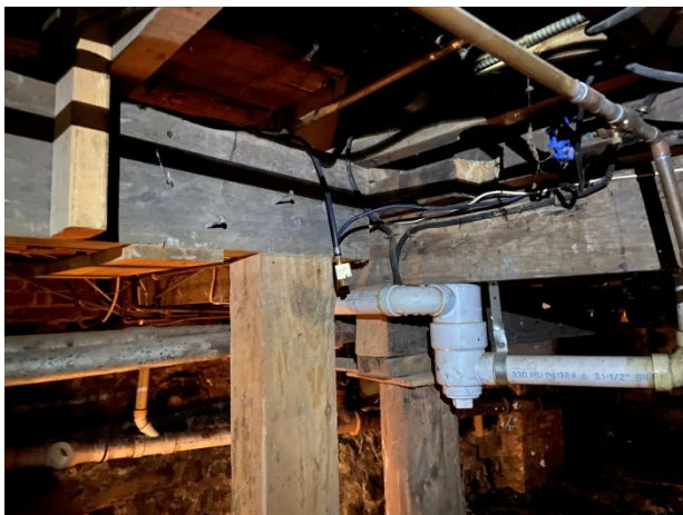
11-First floor framing
