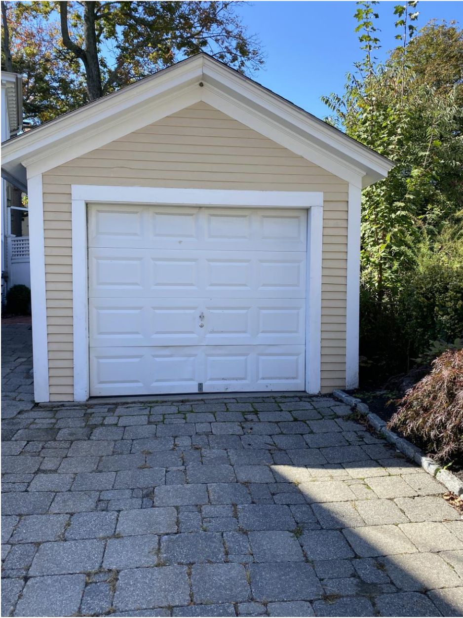
Existing Garage Door:
