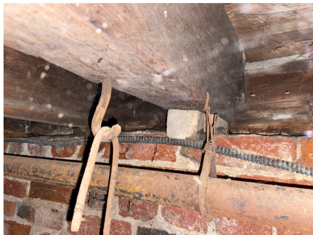
12-Joist supported on shim
