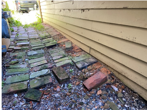
6-Grade along east side
