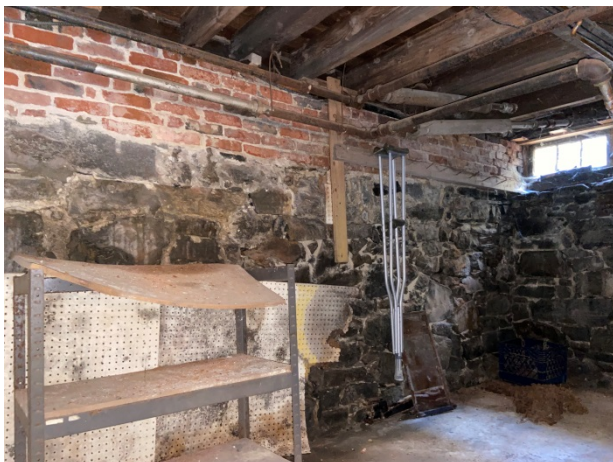
9-View along east side wall
