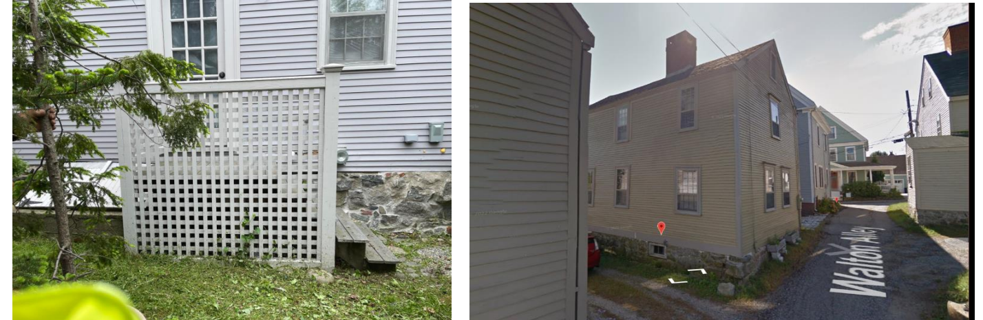
Rear Elevation and Streetscape View
