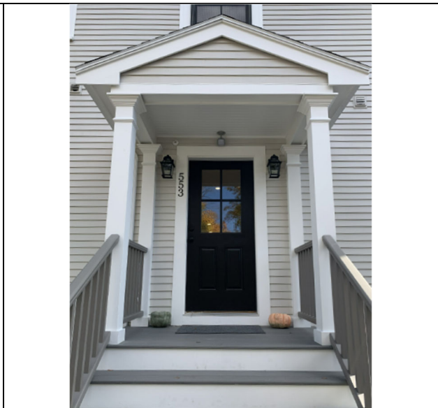
Completed portico – Pilasters added
