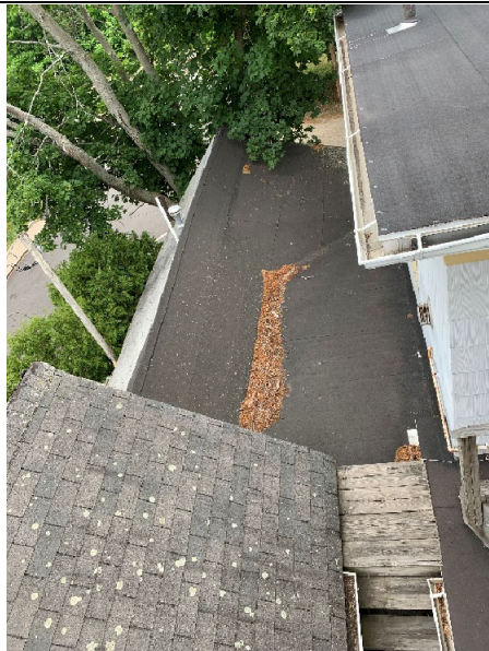
Original low-slope roofs (looking down from above)
