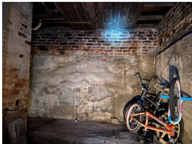
24-Basement looking south
