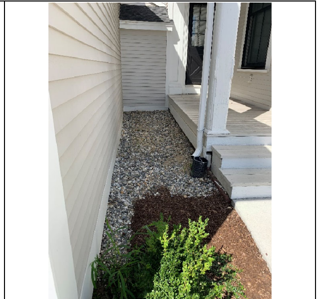
Completed deck – 17" +/- above grade
