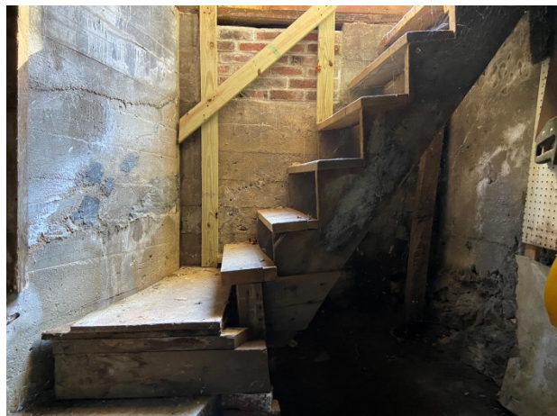
10-Concrete and brick foundation
