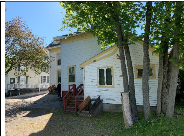
Rear of original side addition
