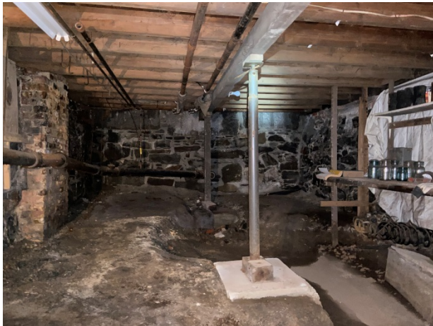
7-Basement looking north
