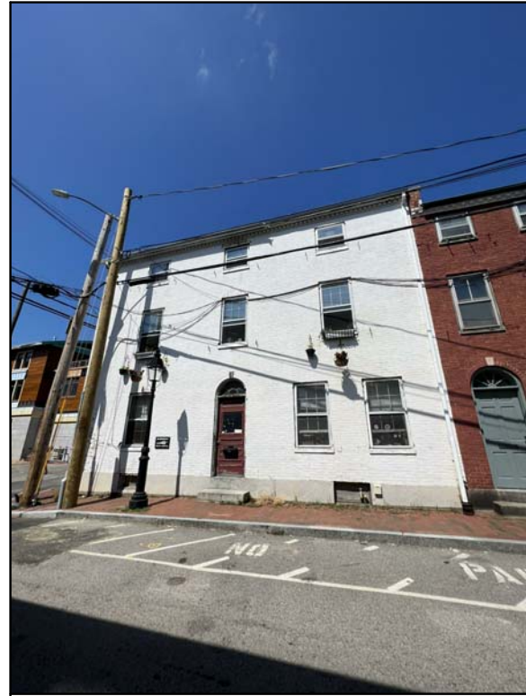
22.) 3 SHEAFE STREET: 26' - 8" (F)
