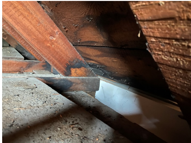
30-Rafter and attic floor joists at eave
