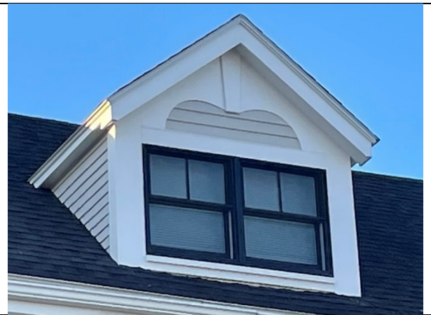
Completed dormer with added trim
