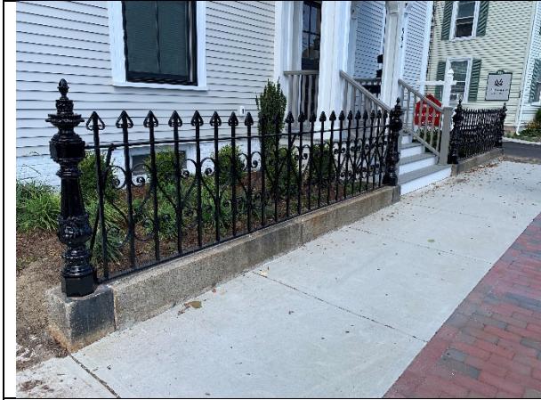
Wrought iron fence repaired
