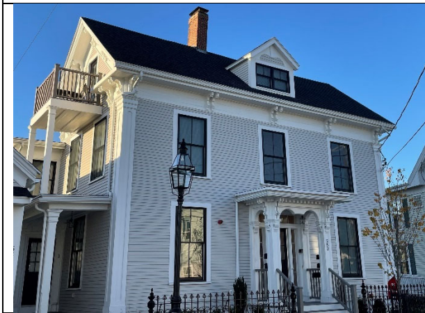
Completed dormer with added trim
