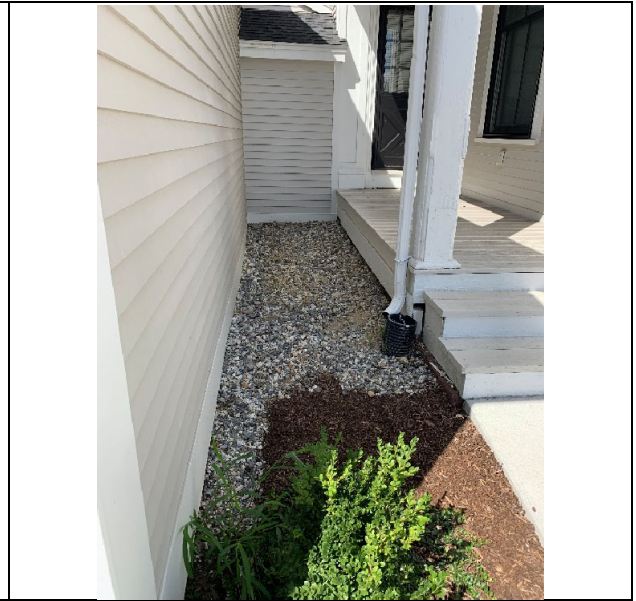
Completed deck – 17" +/- above grade
