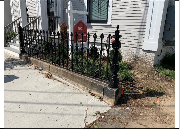
Wrought iron fence repaired
