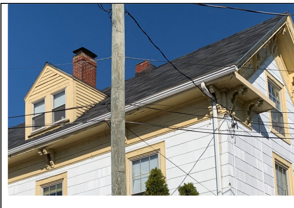
Original chimney, capped at ridge
