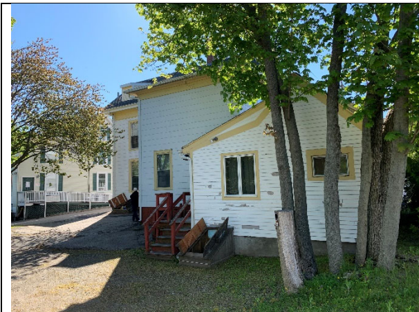
Rear of original side addition
