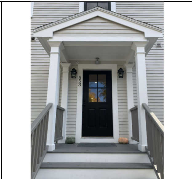
Completed portico – Pilasters added
