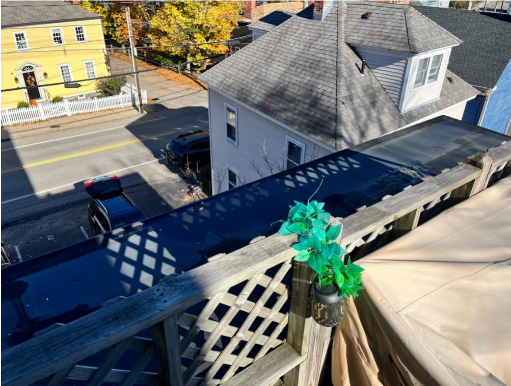
Figure 8. Exposed roof area facing Maplewood.
