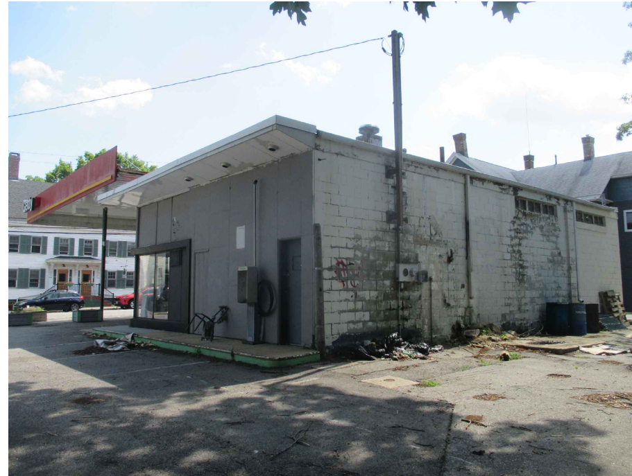
EXISTING NORTH EAST BUILDING CORNER
