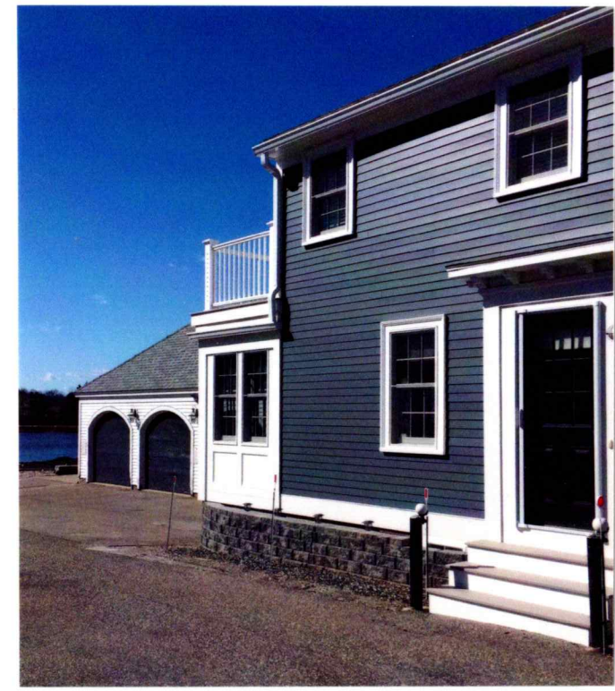
HARD-PLANK LAP SIDING AT EXIST. BUILDING
