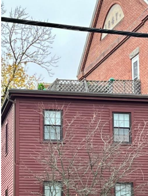
Figure 5. Rooftop perspective as seen from Maplewood street level.
