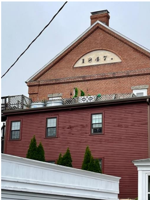
Figure 6. Rooftop as seen from Dennett and adjoining fire escape on left side.
