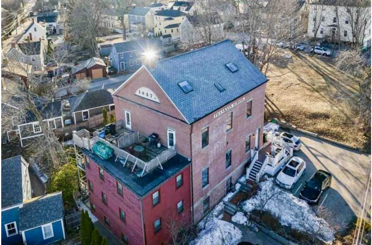
Figure 3. Drone image showing existing rooftop deck configuration including exit doors from Units 4 & 5 and height relative to adjacent homes.
