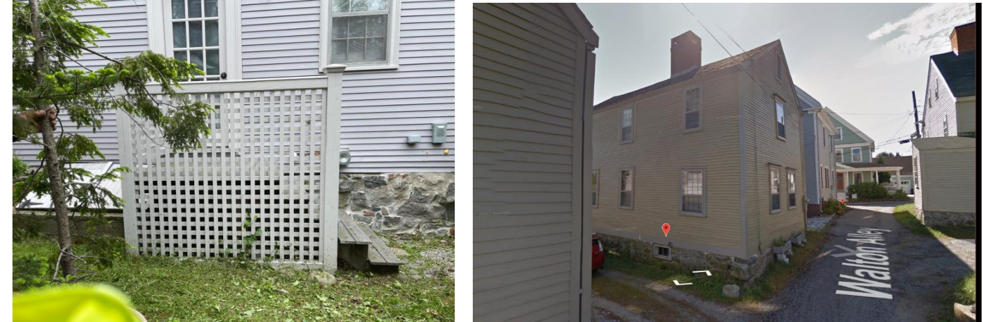
Rear Elevation and Streetscape View
