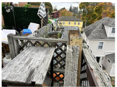
Figure 7. Rooftop as seen facing Maplewood and showing existing railing with lattice and propped vs. secured. Also showing exposed EPDM to edge.
