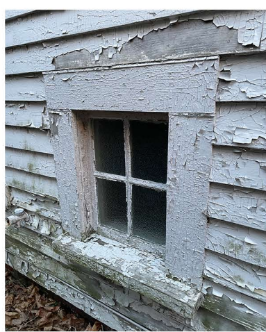
WINDOW SILL NEAR/ON GRADE
