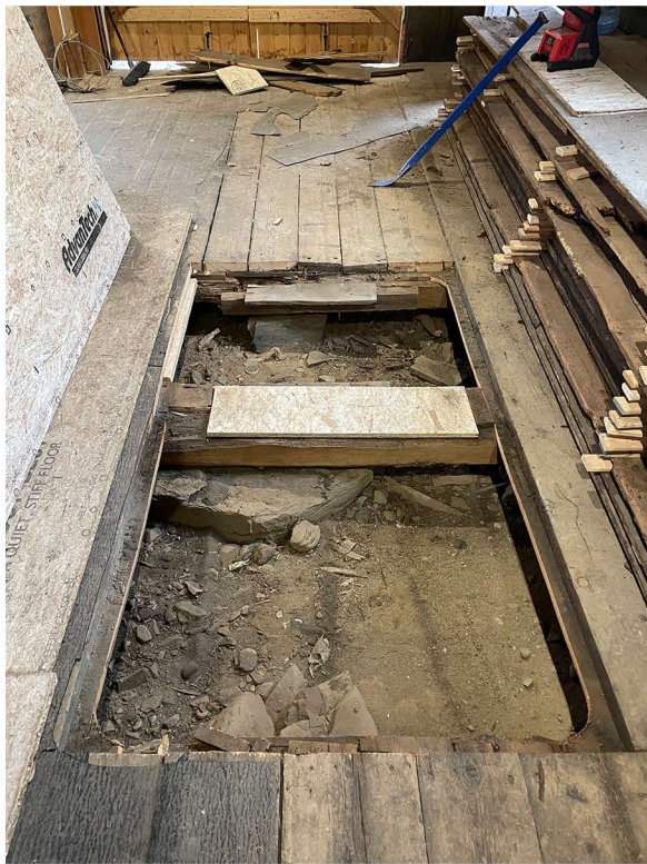
TYPICAL BEAMS IN DIRECT CONTACT WITH GROUND
