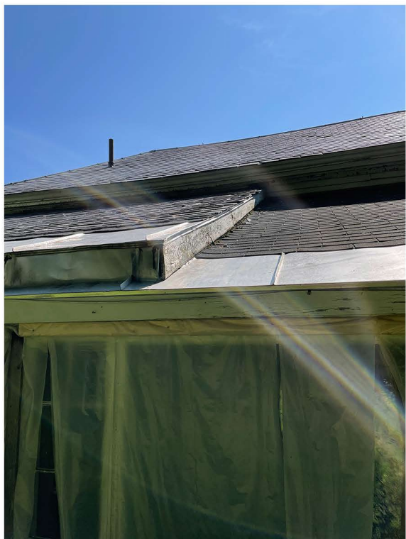
INSUFFICIENT ROOF FLASHING
