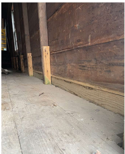
PRESSURE TREATED SILL REPAIR
