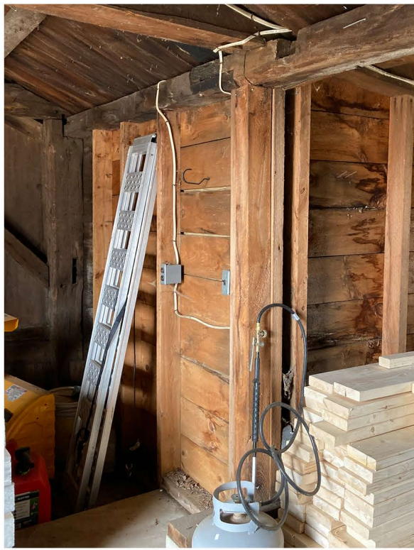
NEW FRAMING AT REAR WALL
