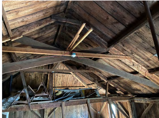
22-Modified roof framing at line 7.5
