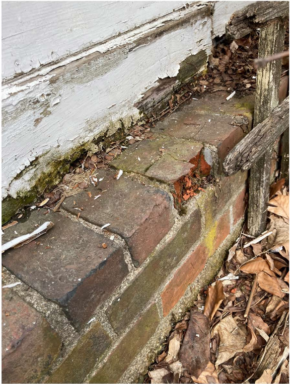
FOUNDATION SHELF AND ROT FROM STANDING WATER
