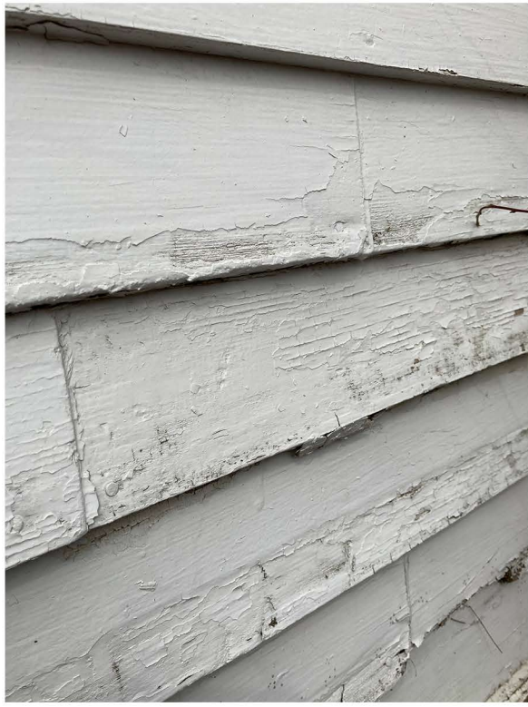
TYPICAL SIDING BUTT JOINT
