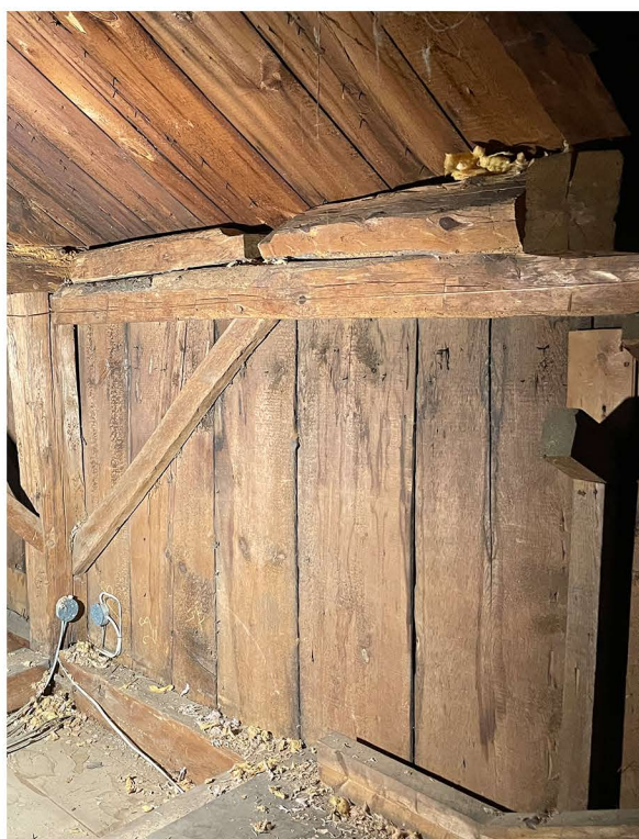
OLDER FRAMING MEMBERS HAVE BEEN MODIFIED, REMOVED, OR RELOCATED. (SECOND FLOOR OF CARRIAGE HOUSE)
