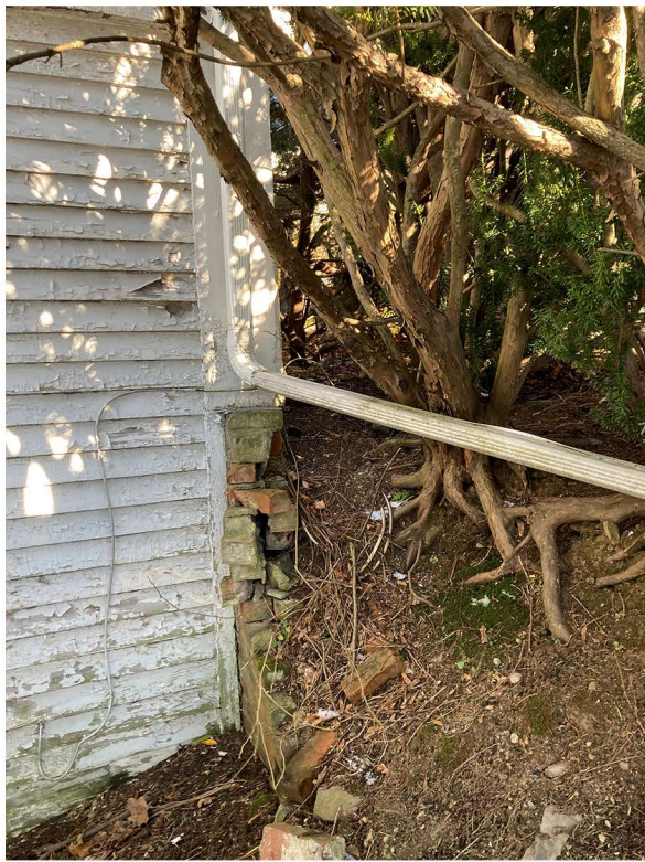
CRUMBLING FOUNDATION LACKING POSITIVE DRAINAGE
