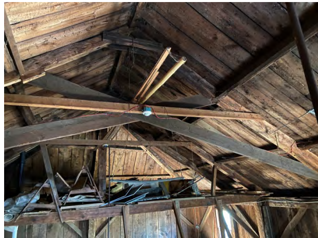
22-Modified roof framing at line 7.5
