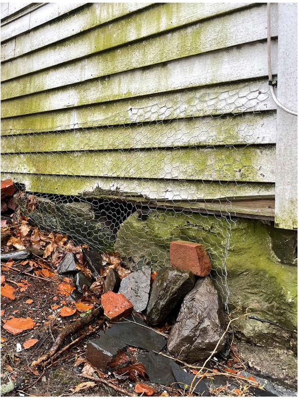
STONE RUBBLE FOUNDATION AND NEW SIDING REPAIR
