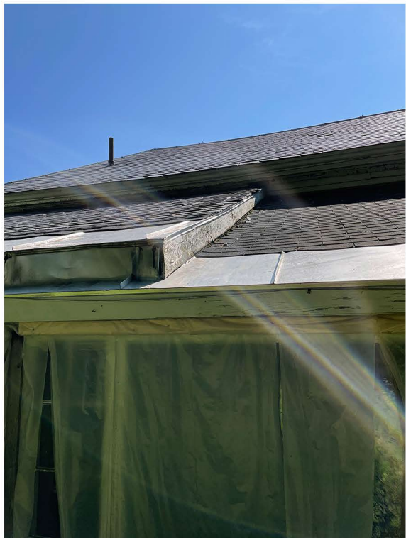
INSUFFICIENT ROOF FLASHING
