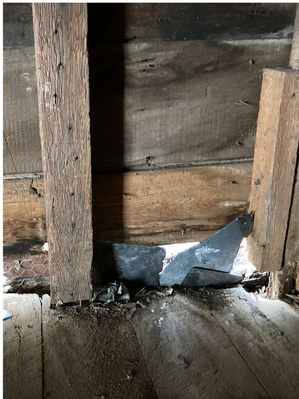
COMPROMISED STRUCTURE AT BASE
