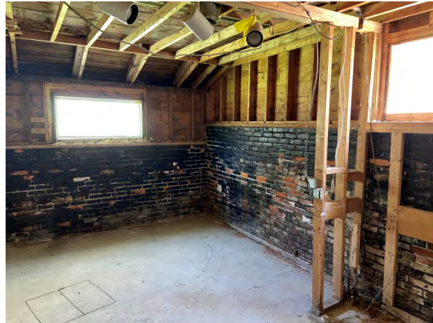
20-Brick foundation and side wall framing
