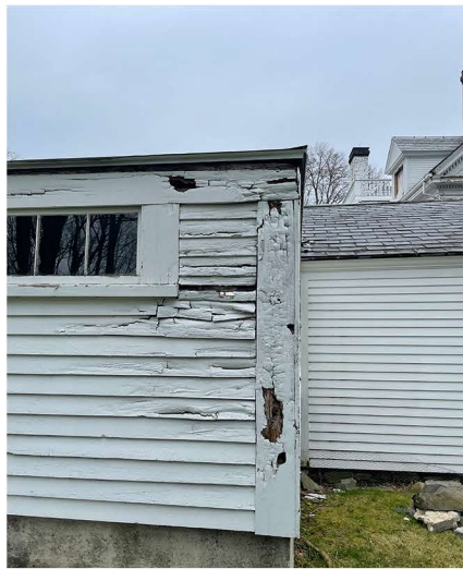
SIDING / CORNER BOARD ROT
