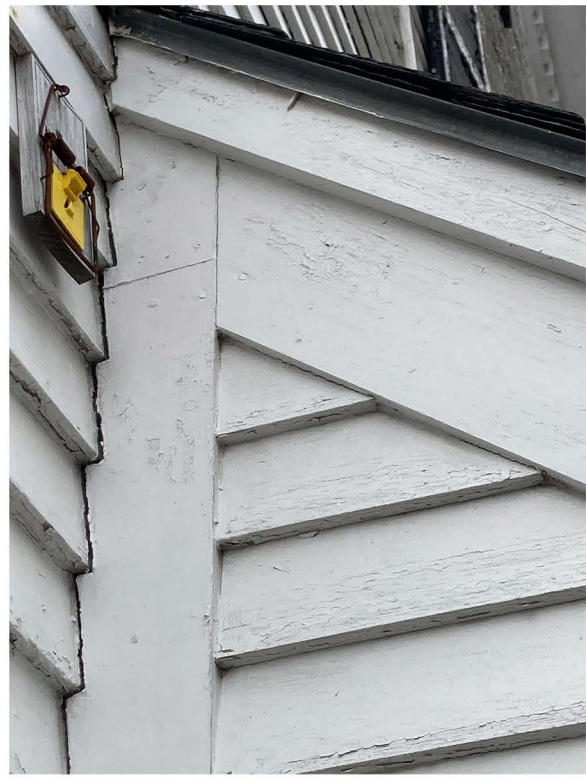
CORNER BOARD NOTCHED AGAINST ANNEX SIDING
