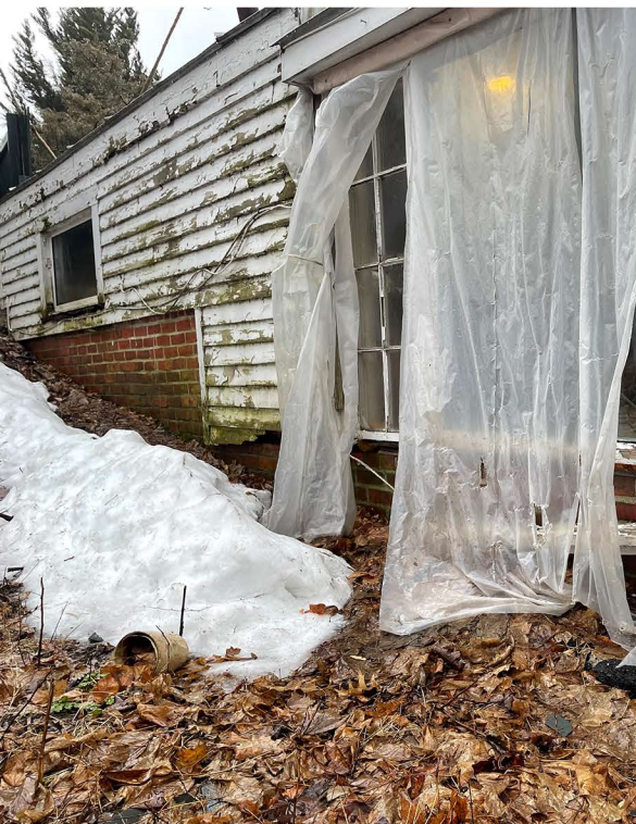
TYPICAL SIDING ROT AND FOUNDATION DAMAGE
