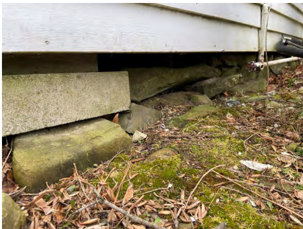
5-Connector foundation on north side
