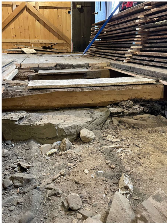
TYPICAL BEAMS IN DIRECT CONTACT WITH GROUND
