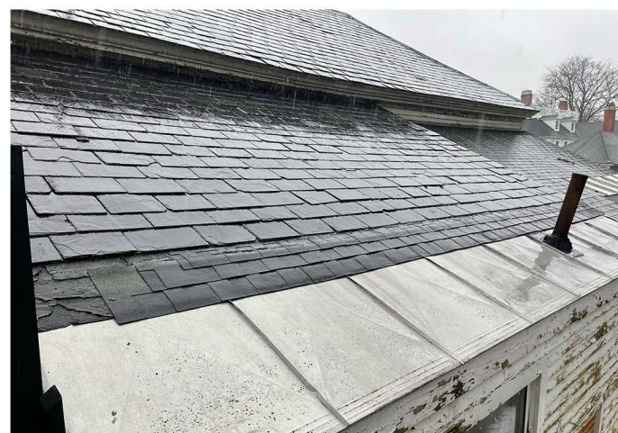
SLATE, ASPHALT AND, METAL ROOFING
