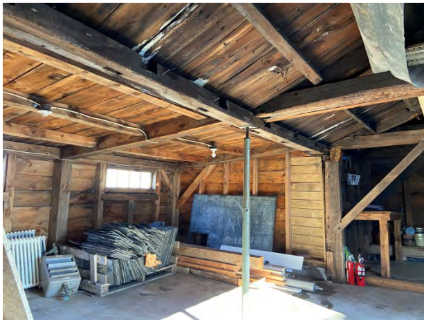
13-5x5 timber supported on screw jack
