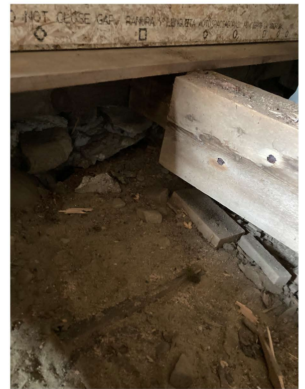
TYPICAL FLOOR FRAMING MADE UP OF REPURPOSED BEAMS
