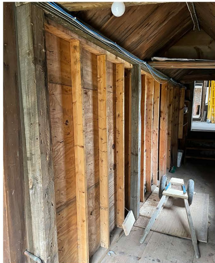
INTERIOR STUDS / PLYWOOD
