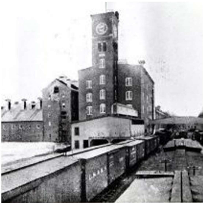
88 MAPLEWOOD (LOT 5) PORTSMOUTH, NEW HAMPSHIRE
