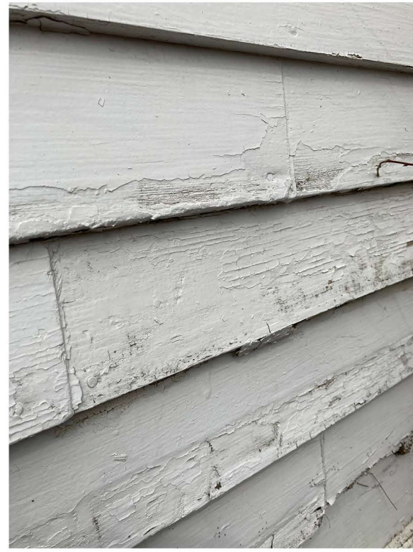
TYPICAL SIDING BUTT JOINT
