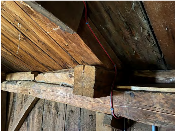
21-Cut bottom chord on line 7.5
