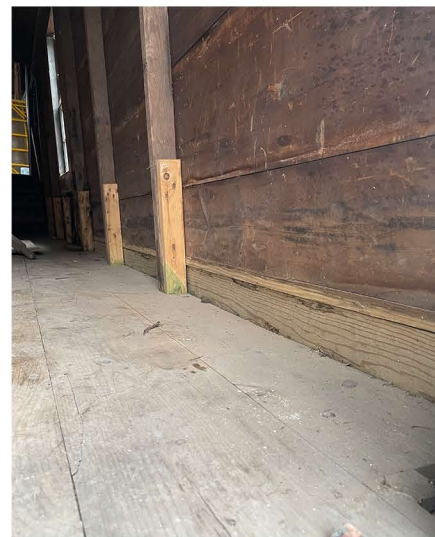
PRESSURE TREATED SILL REPAIR
