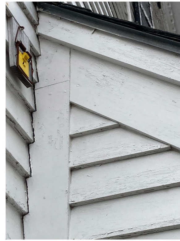
CORNER BOARD NOTCHED AGAINST ANNEX SIDING
