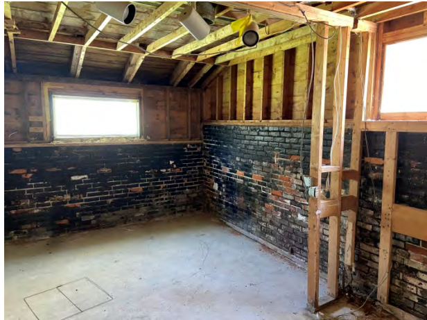
20-Brick foundation and side wall framing
