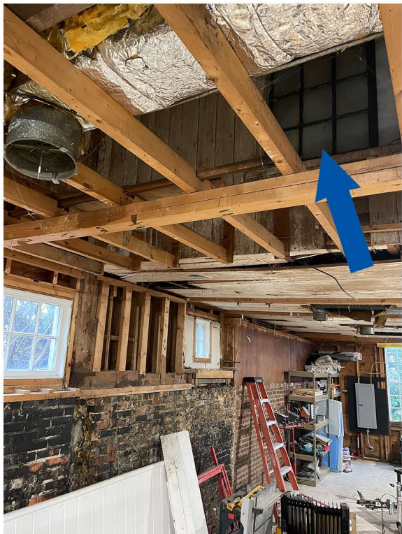
EXISTING WINDOW LOCATED AT REAR OF ORIGINAL CARRIAGE HOUSE BLOCK
