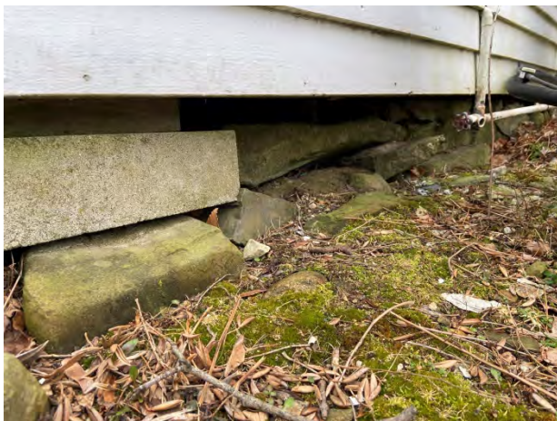
5-Connector foundation on north side
