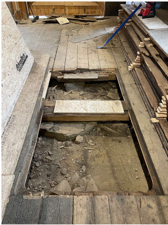
TYPICAL BEAMS IN DIRECT CONTACT WITH GROUND
