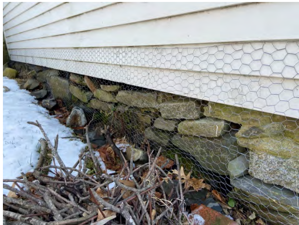
10-Stone foundation along back of barn
