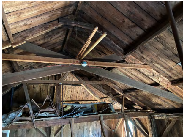
22-Modified roof framing at line 7.5
