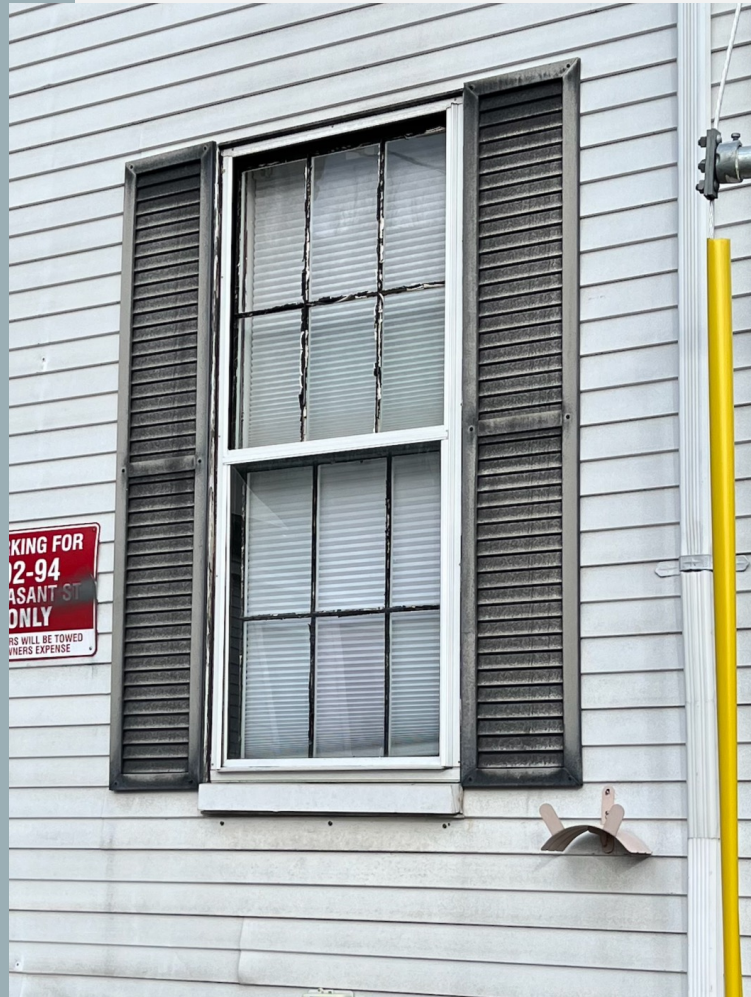
Existing sash and storms
