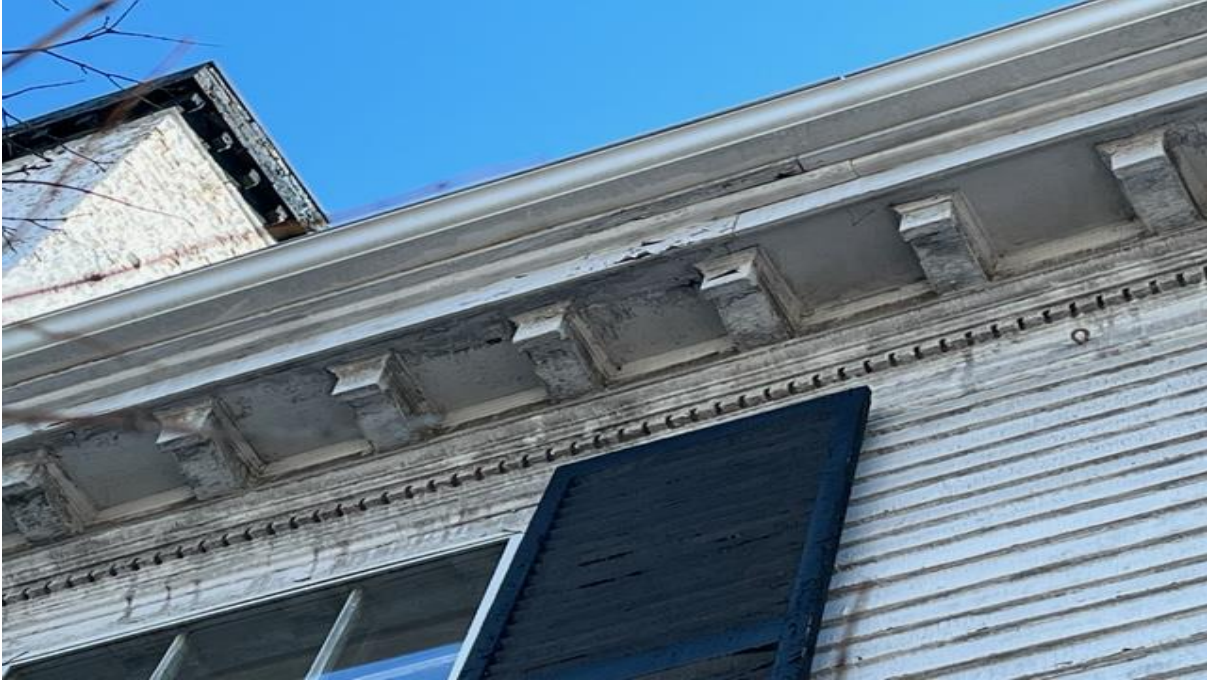
North wall with water issues, cornice repair
