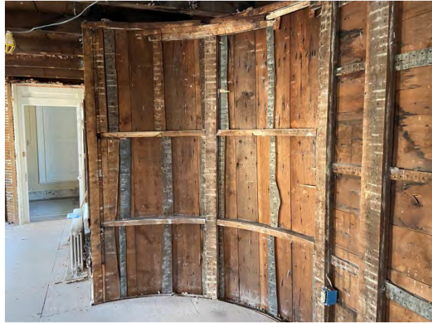
Curved wall framing as second floor
