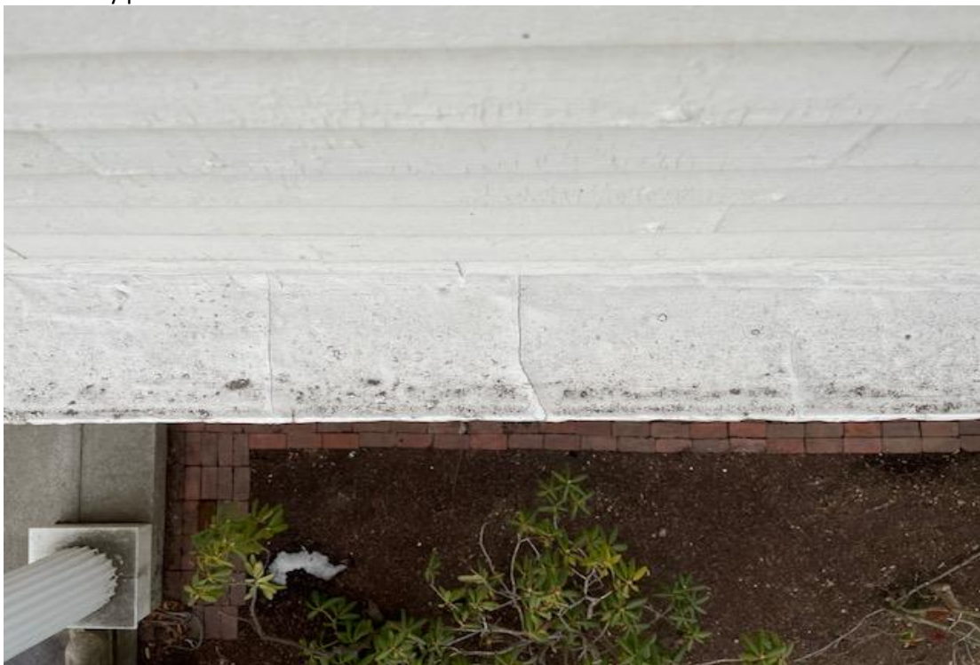
Window head unit flashing
