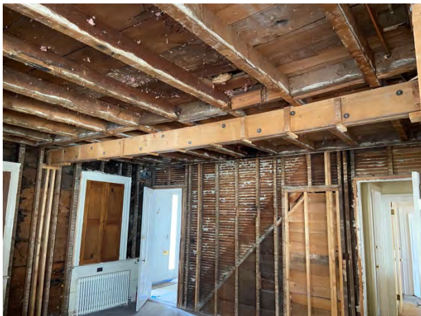
(4)2x10 beam at supporting second floor
