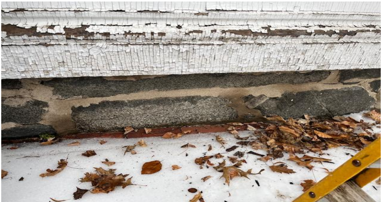
Existing foundation stone, square and rectangular granite slabs
