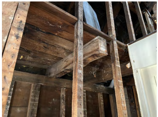
Annex third floor unsupported framing
