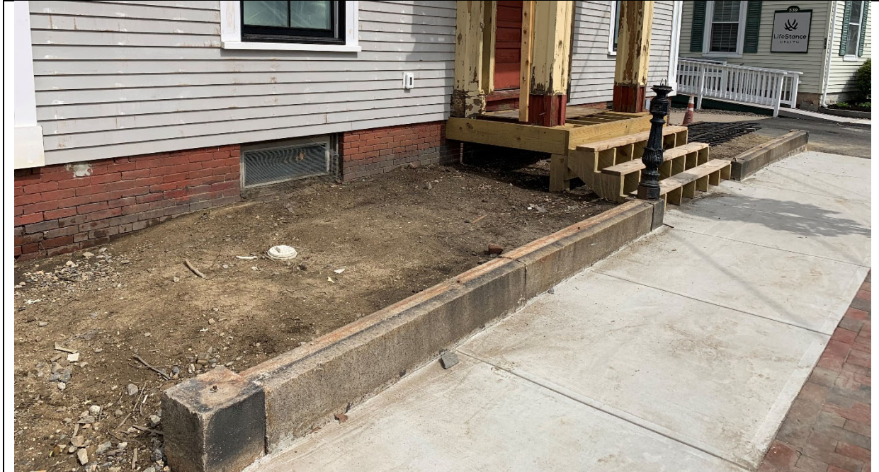
Current conditions (under construction) – Railing removed, granite curb removed and reset by City (Severino) for sidewalk and sewer connection
