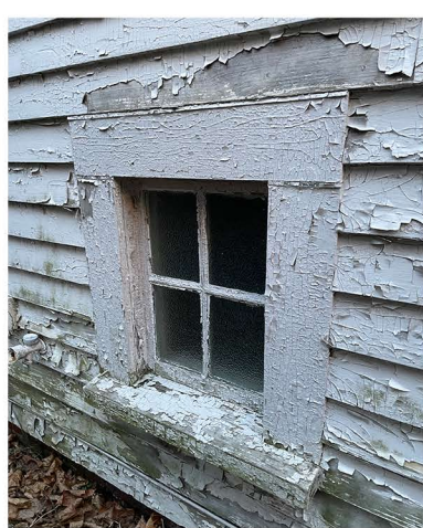
WINDOW SILL NEAR/ON GRADE
