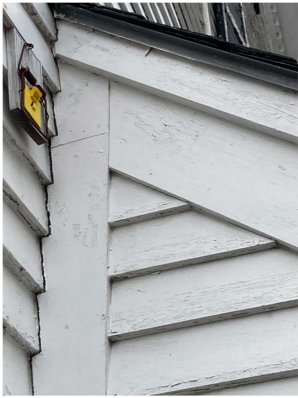
CORNER BOARD NOTCHED AGAINST ANNEX SIDING
