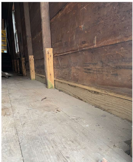
PRESSURE TREATED SILL REPAIR
