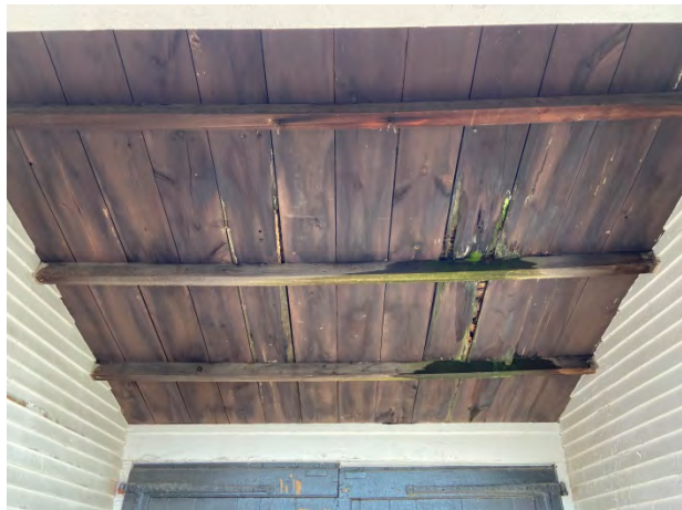
14-Connector roof sheathing and purlins
