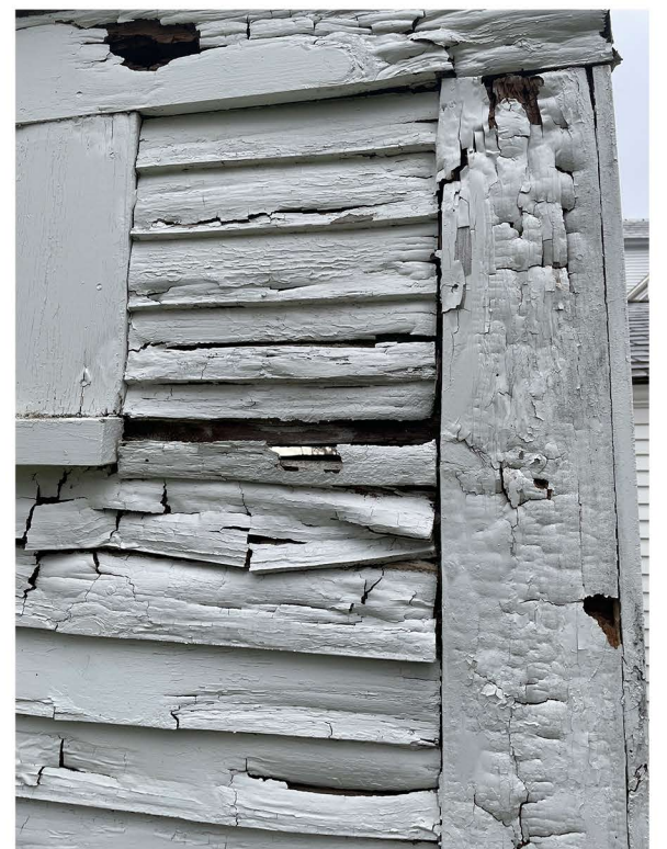
SIDING ROT AND INSUFFICIENT FLASHING
