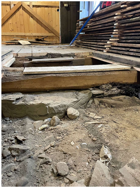
TYPICAL BEAMS IN DIRECT CONTACT WITH GROUND
