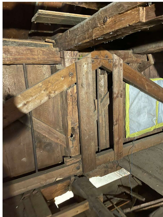
OLDER FRAMING MEMBERS HAVE BEEN MODIFIED, REMOVED, OR RELOCATED. (SECOND FLOOR OF CARRIAGE HOUSE)
