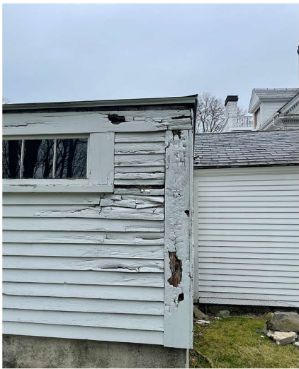
SIDING / CORNER BOARD ROT
