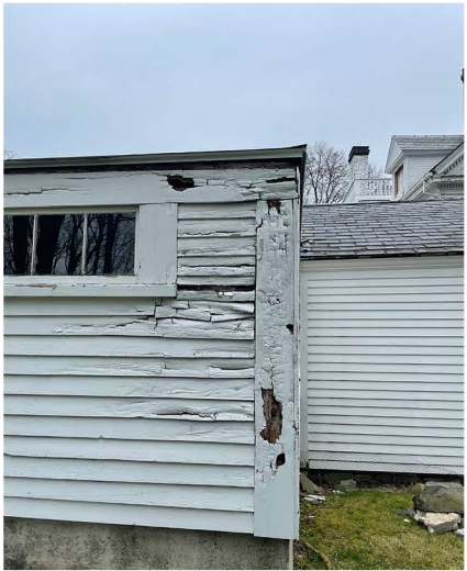
SIDING / CORNER BOARD ROT
