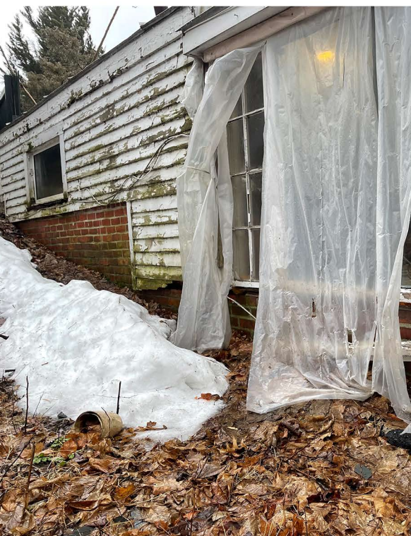
TYPICAL SIDING ROT AND FOUNDATION DAMAGE
