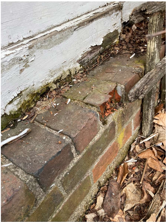
FOUNDATION SHELF AND ROT FROM STANDING WATER
