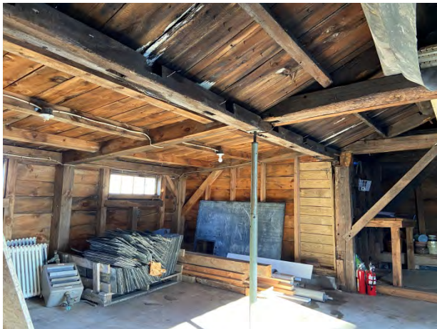
13-5x5 timber supported on screw jack
