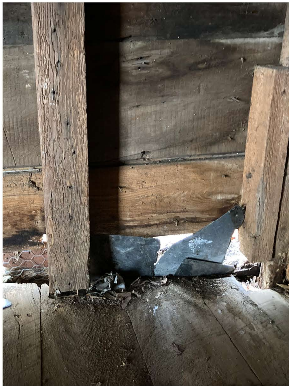
COMPROMISED STRUCTURE AT BASE
