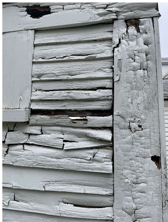
SIDING ROT AND INSUFFICIENT FLASHING
