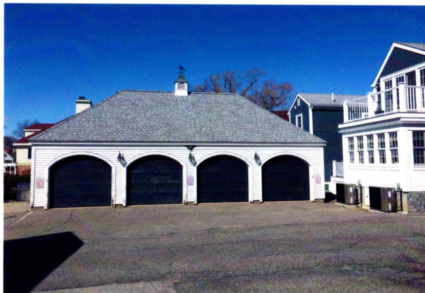
EXISTING GARAGE SOUTH VIEW
