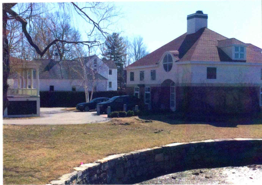
VIEW FROM NORTH MILL POND BRIDGE
