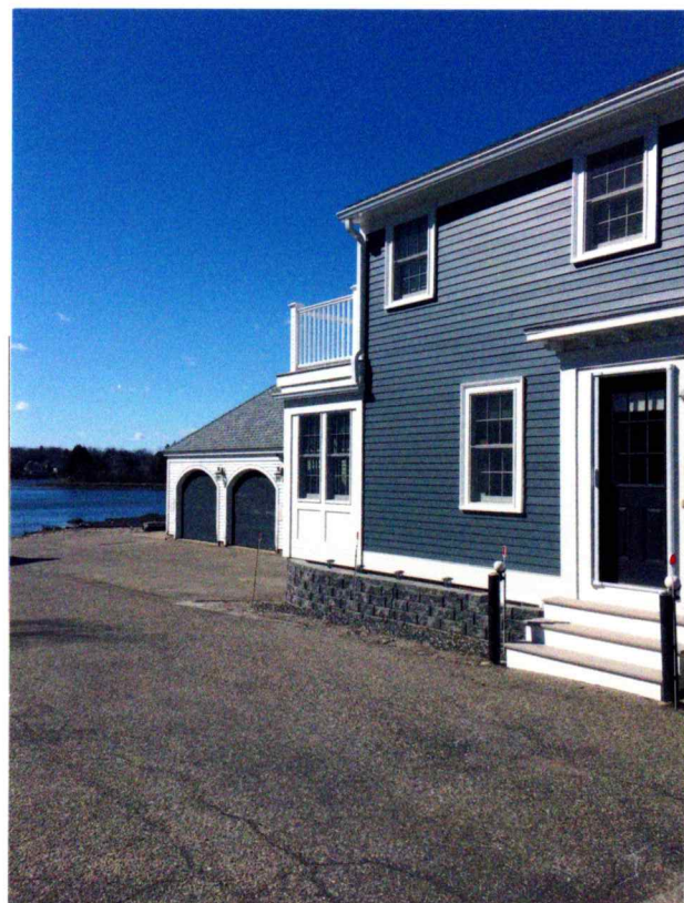
VIEW FROM DRIVEWAY ENTRY
