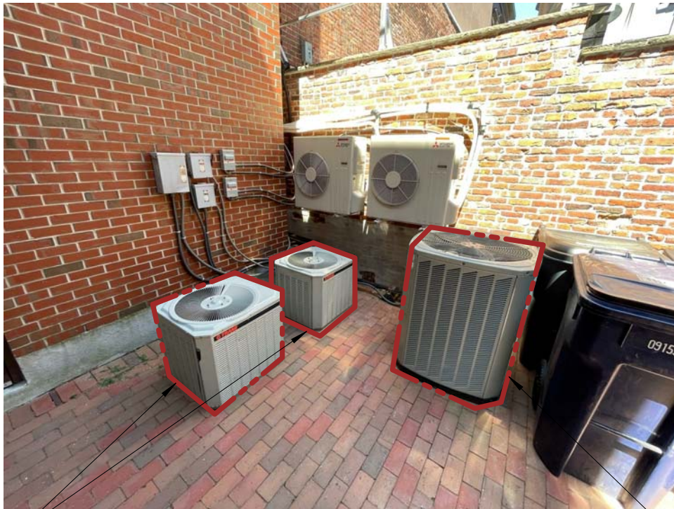
ALL EXISTING GROUND MOUNTED CONDENSER UNITS (3) TO BE REMOVED, REFER TO SHEET SKH-1
