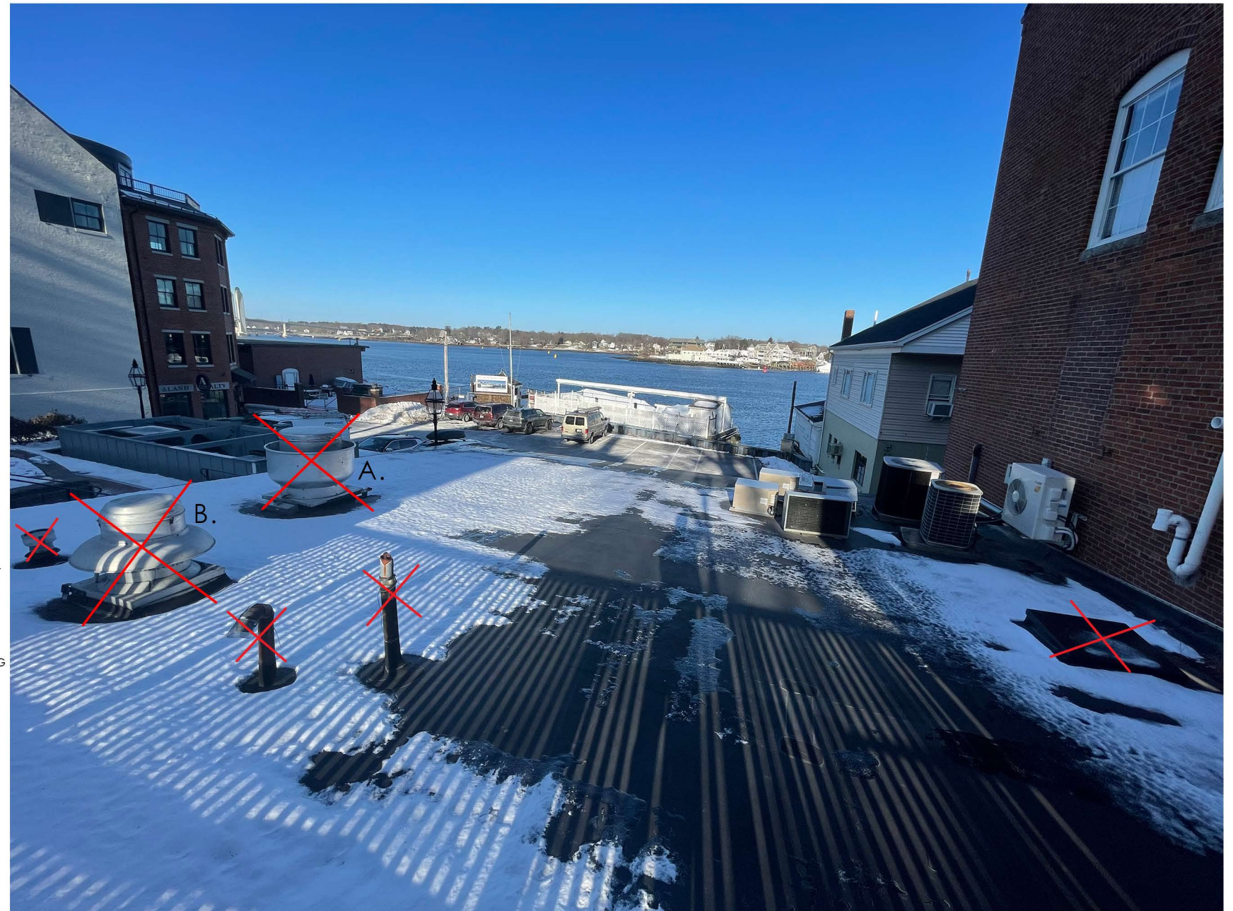
EXISTING RESTAURANT INTAKE AND EXHAUST FAN DIMENSIONS A: 42"H x 44"W (10" CURB HEIGHT) B: 33"H x 33"W (9" CURB HEIGHT)
