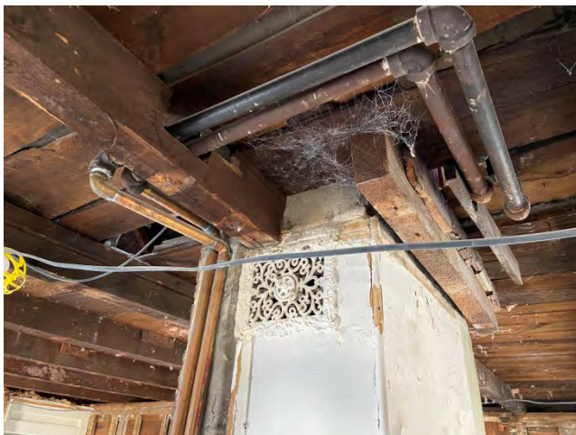
Third floor framing supported at chimney
