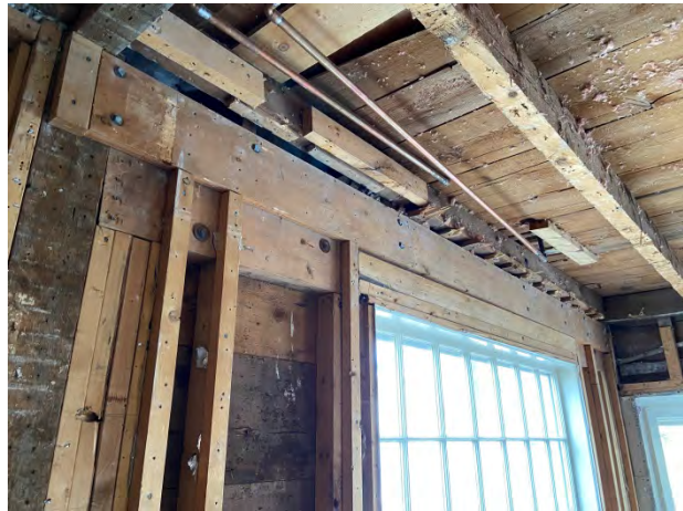
Wall framing at window
