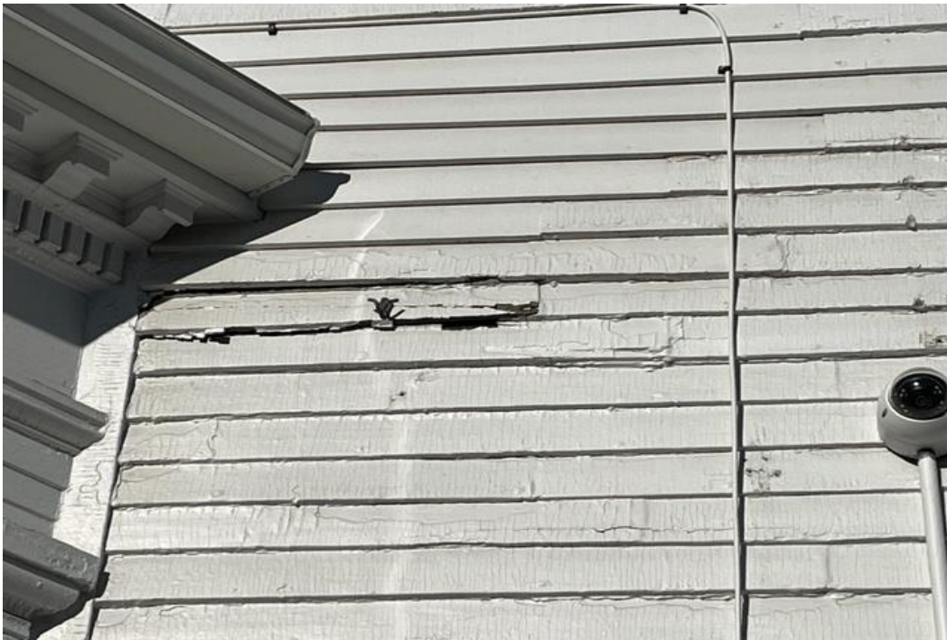
Siding & Trim repair/replacement
