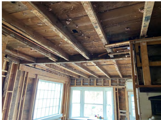
3"x7½" beam supporting second floor
