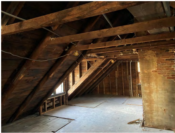
Roof framing at dormer
