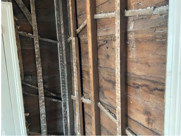
3x3 and 2x2 first floor wall framing
