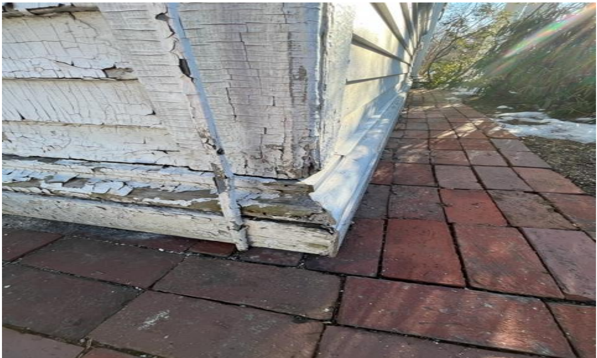
Bricks and grade at or above sill beam, promoting rot
