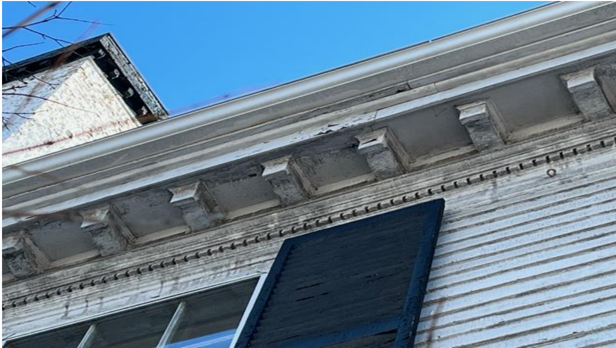
North wall with water issues, cornice repair
