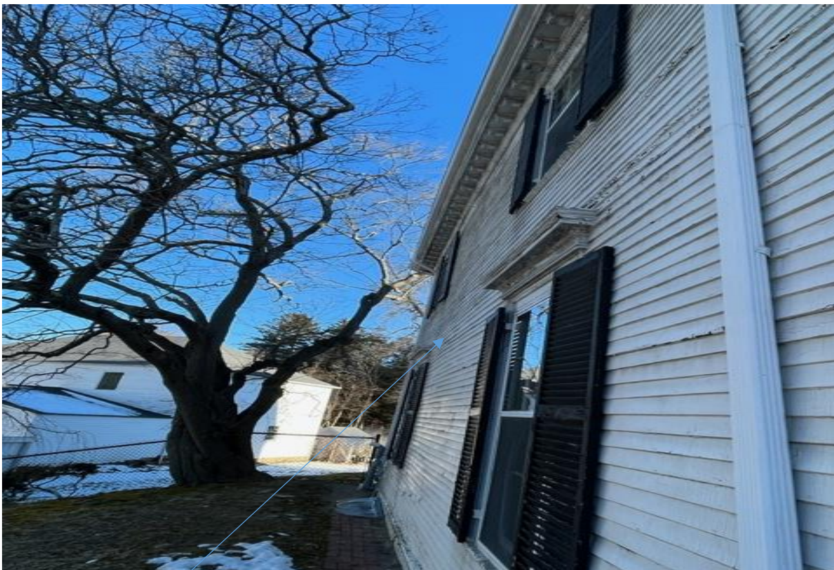
North wall with water issues, significant bow in wall
