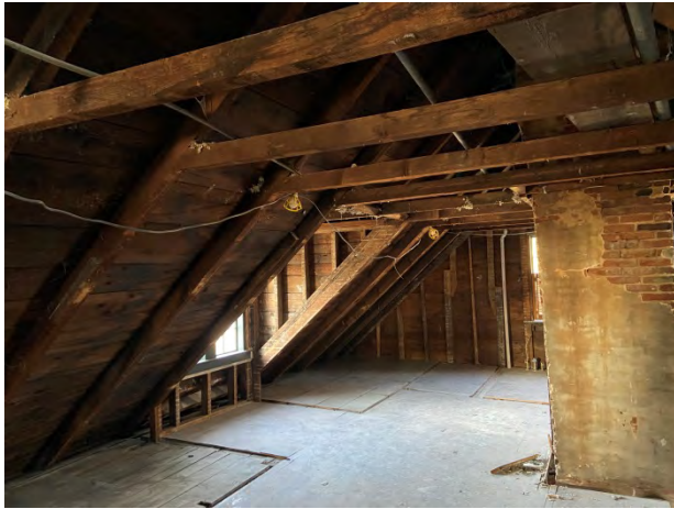
Roof framing at dormer
