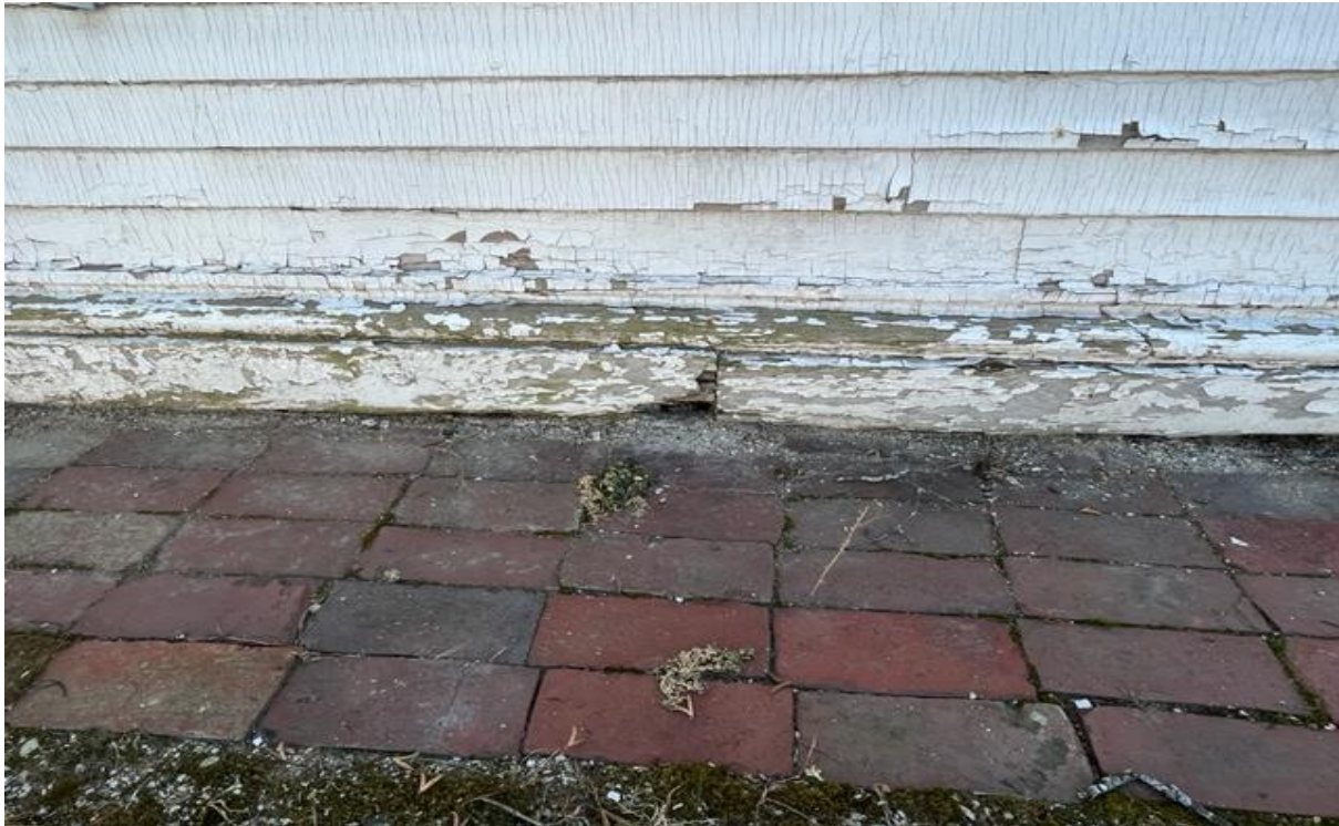
Bricks and grade at or above sill beam, promoting rot
