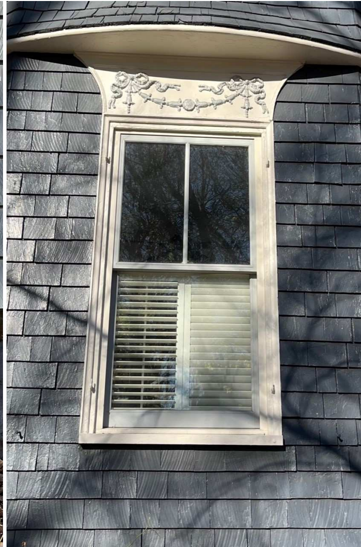
Window Trim Casing and Sill
