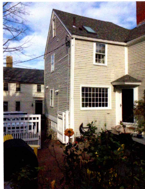
VIEWS OF REAR ELEVATIONS
