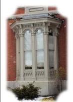
3. Sash and jamb liner track applications: With this system we make new energy efficient sash that mimic the sightlines of the original sash. And we supply a vinyl jamb liner / sash balance system that gets applied to the existing window frame. Typically the daylight
