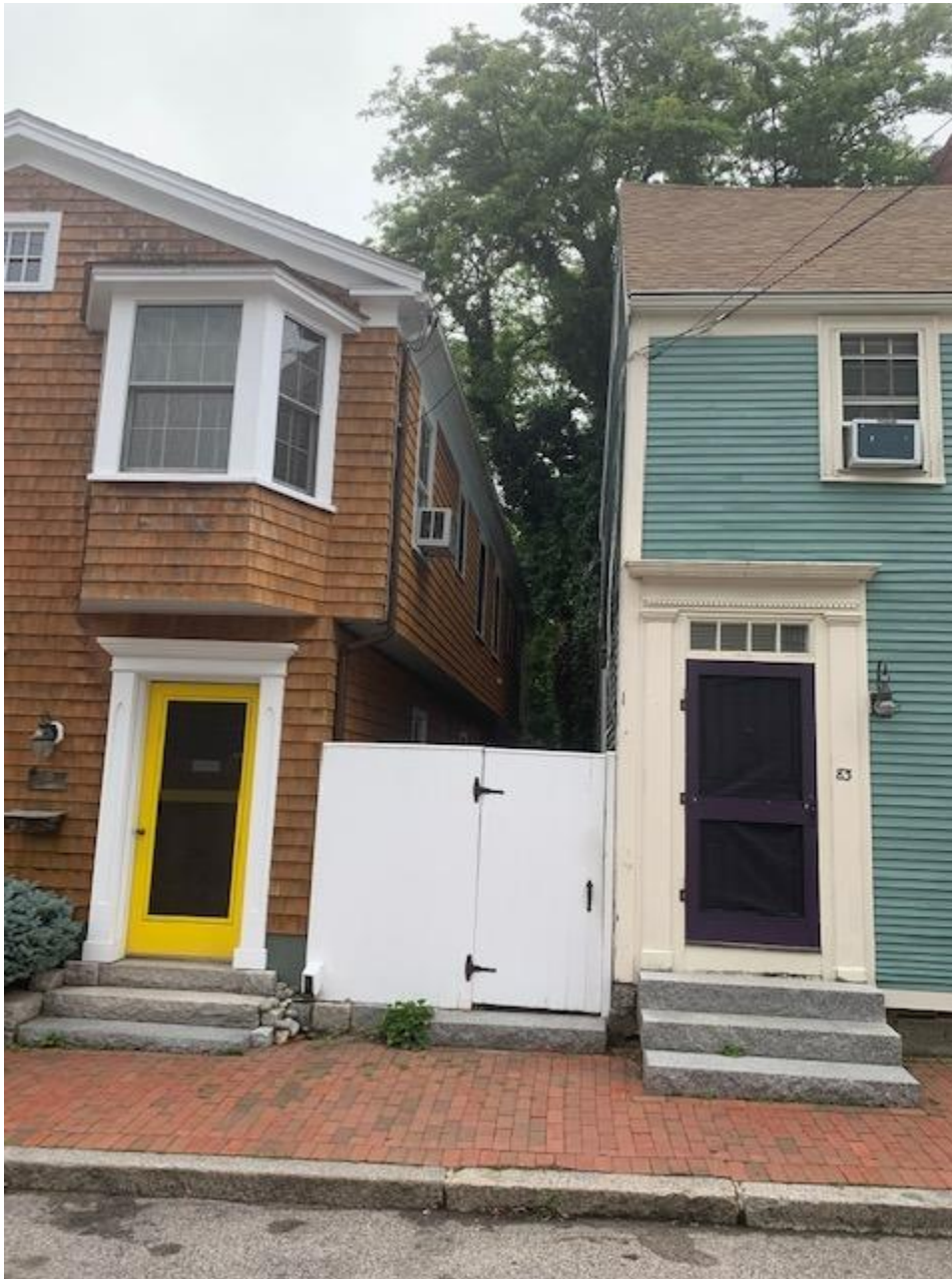
Existing Cedar shingles- proposed to switch to cedar clapboards.
