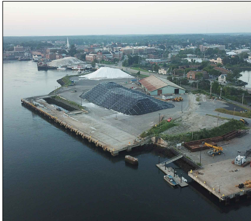
OVERALL SITE LOOKING SOUTH
