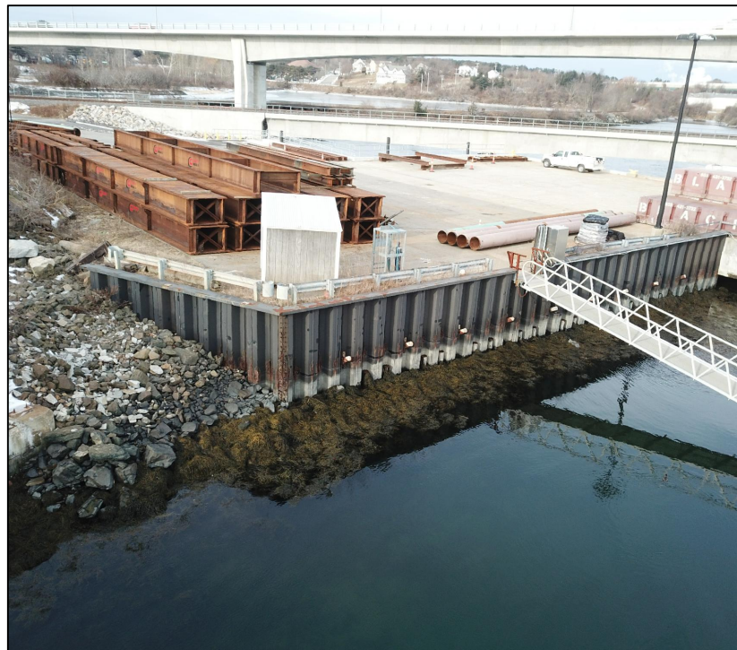
BARGE WHARF BULKHEAD LOOKING WEST (A1)
