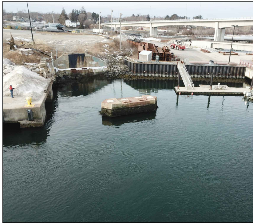
NORTH WHARF EXTENSION LOCATION LOOKING SOUTHWEST (C1)
