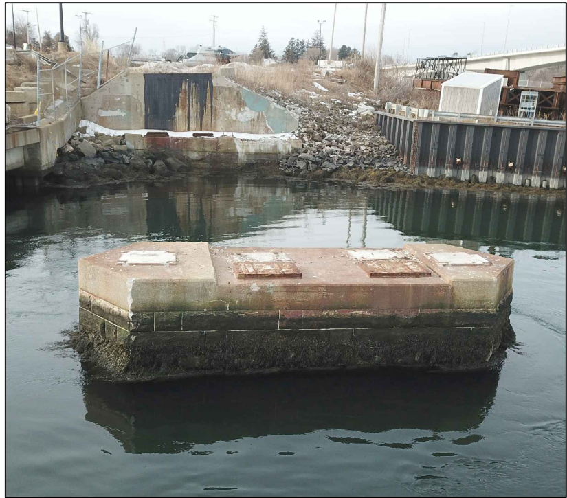
BRIDGE PIER 14 LOOKING SOUTHWEST (C3)
