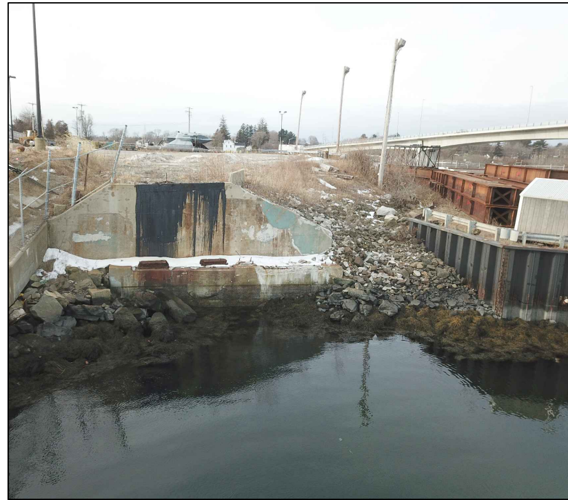
BRIDGE ABUTMENT 13 LOOKING SOUTHWEST (C4)
