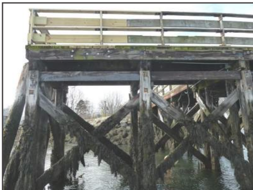
11. T-Head pier Recent repair from arson event. It is estimated that the T-Head Pier has 20 years of service life remaining, assuming it is repaired and maintained.
