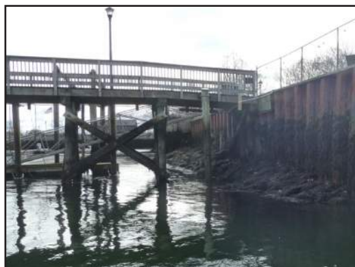
21. North Pier It is recommended to replace the timber bracing as soon as possible.
