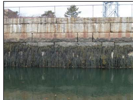
16. Quaywall Repointing existing block.
