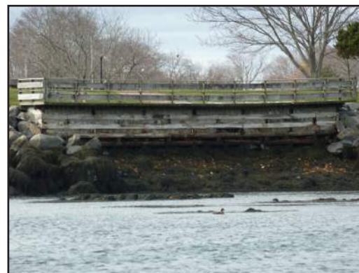
24. Four Tree Island Deck with missing rip rap and erosion undermining structure along east shore.
