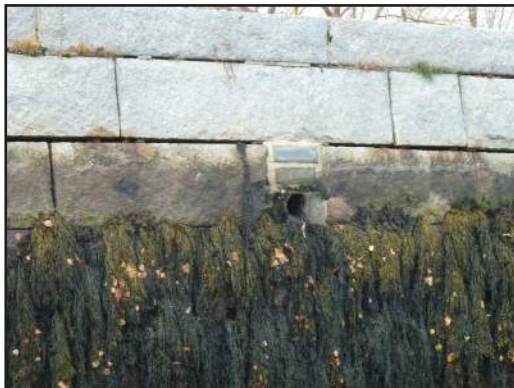
15. Quaywall Stromwater out fall.
