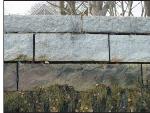
14. Quaywall Repoint and mortar joints.
