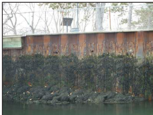
19. At north pier Steel is deteriorating with significant pitting with visible holes at high tide line.
