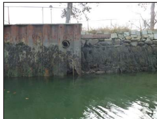
20. Steel bulkhead Significant settlement and slumping visible. Wall requires reconstruction.
