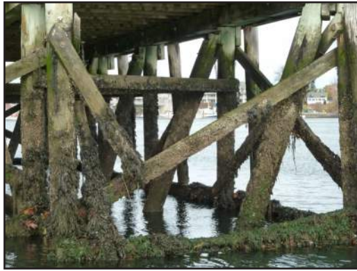
7. South pier Broken cross members under deck, it is recommended to replace the failed bracing member as soon as possible. The structure has 15 years of service life remaining, assuming it is repaired and maintained.
