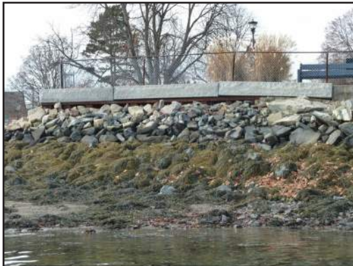
9. Adjacent to T-Head pier Steel sheeting with granite coping and placed rip rap armoring.
