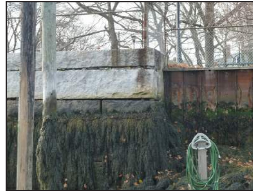
18. From quaywall to steel bulkhead Transition to steel sheeting. Estimated age 20 years.
