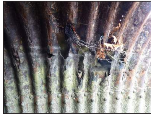
26. Four Tree Island Culvert under causeway requires lining or reinforcement. Excessive section loss in areas.
