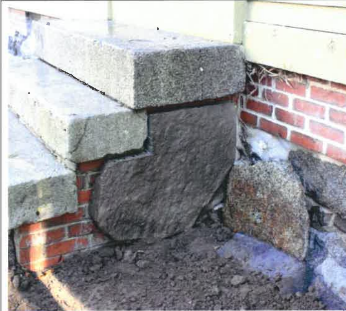
INSERT #34 For purposes of demonstration, re-purposed flagstone was cut to fit, and dry-laid to over existing brick on staircase 2
