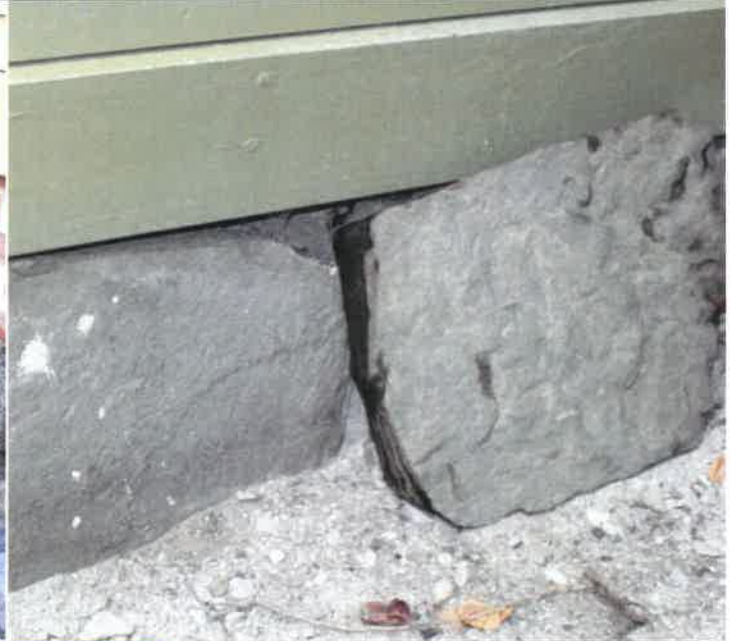
INSERT #35 Flagstone sample put next to existing foundation
