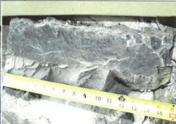
INSERT #25 original blue stone in right side (West) foundation
