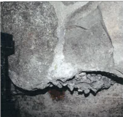
INSERT #41 Existing stone veneer, with mortar visible
