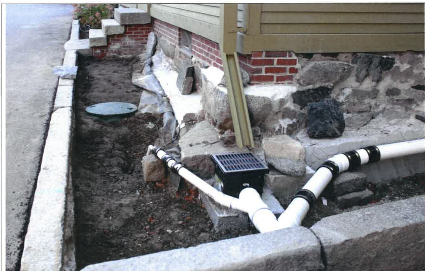
INSERT # 4 Completed roof rainwater drainage system & green catch basin cover for French drain-type system under future front (North) and side (West) garden
