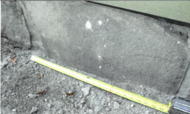
INSERT #24 Large existing flag stone in right side (West) foundation
