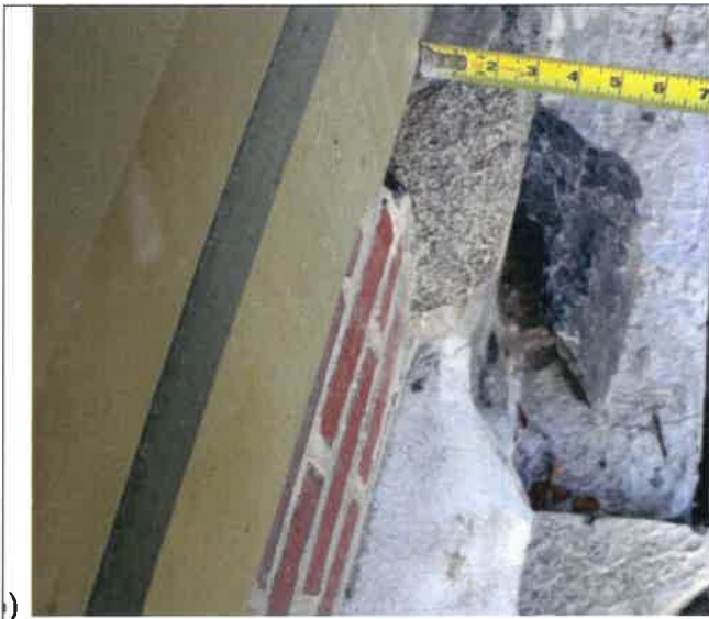
INSERT 56 protruding foundation stone.
