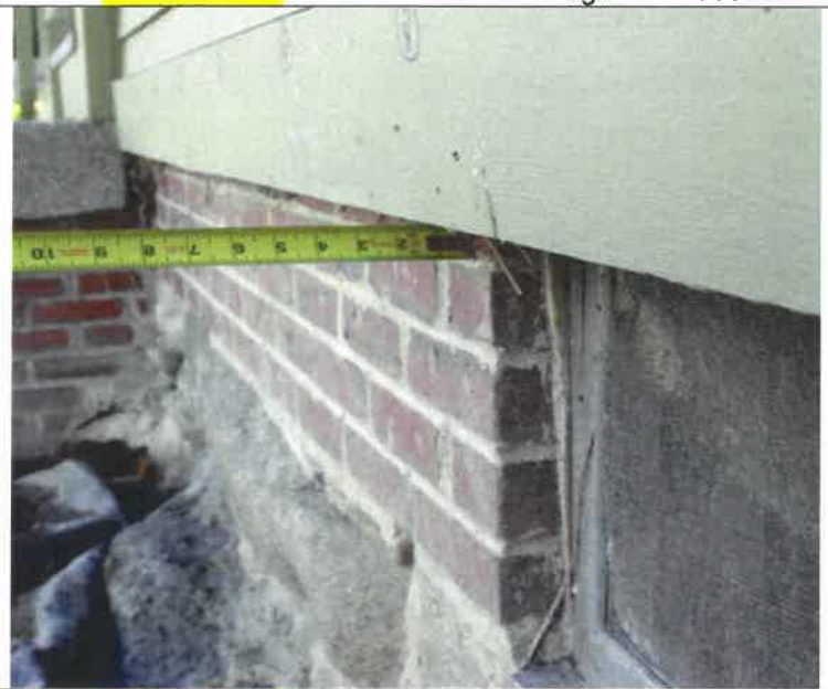
INSERT #54 Waterboard at front right of house
