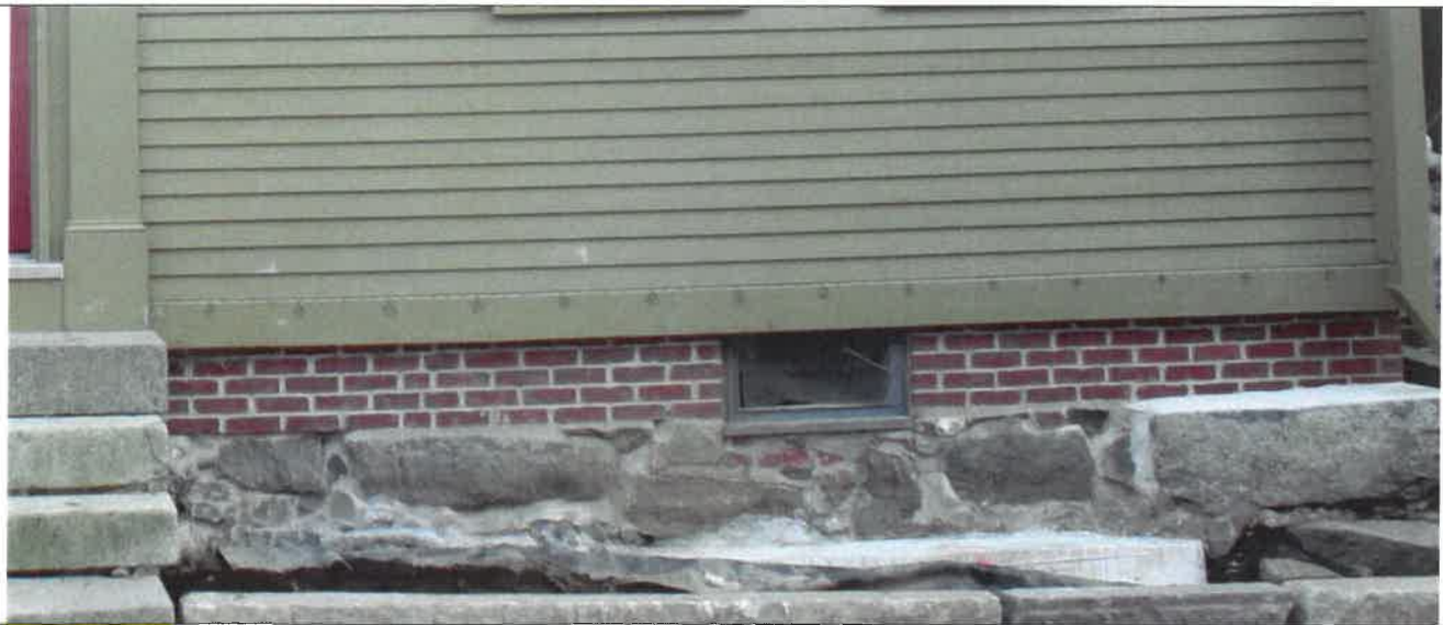
INSERT #21 Front foundation with mostly large stones, primarily granite, of various color, shape & size
