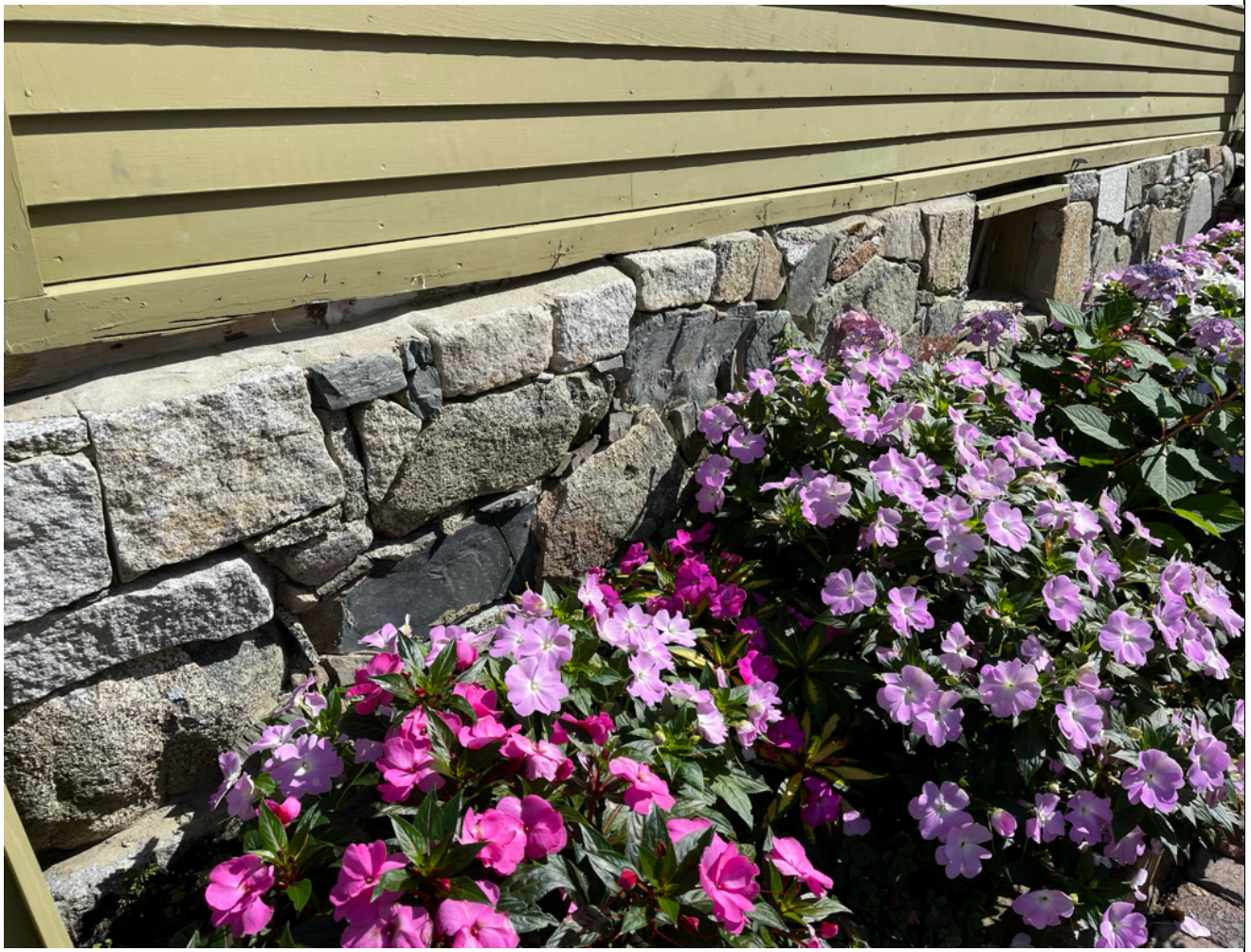
Exhibit-5 (current foundation and under-sized water table trim board. (See also Exhibit-4 above)
