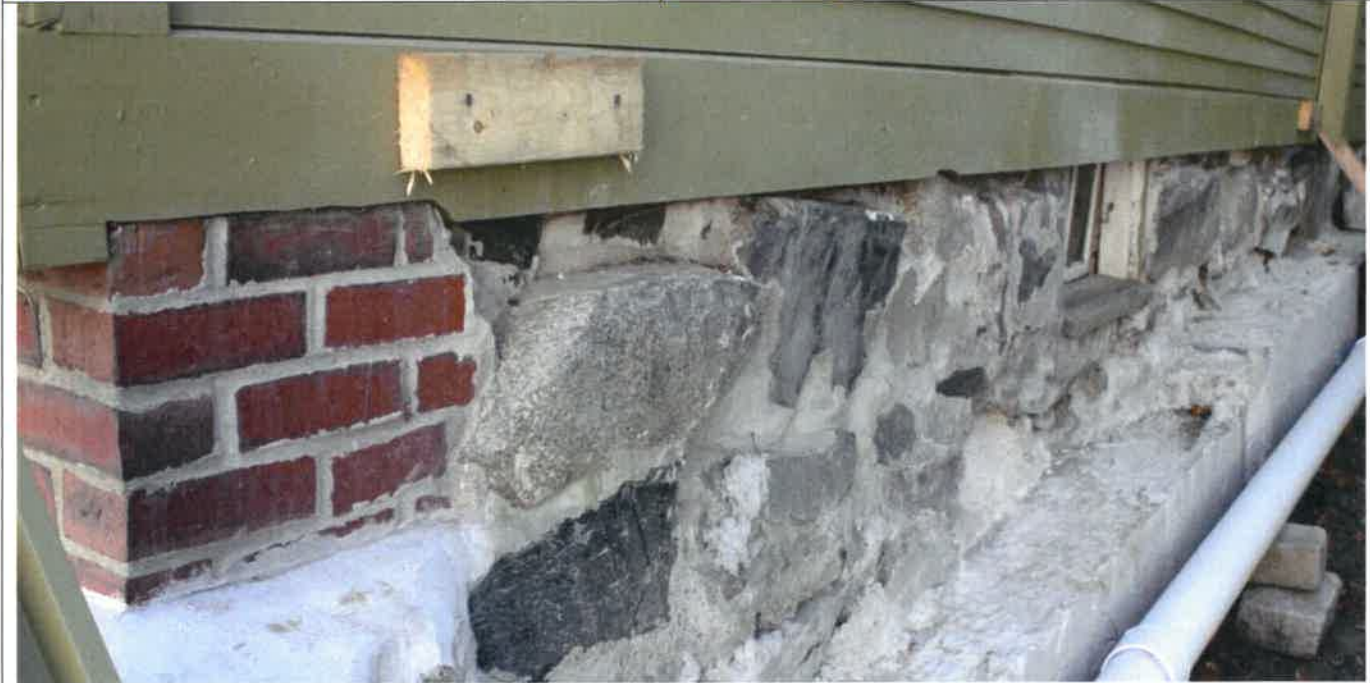
INSERT 56 protruding foundation stone.
