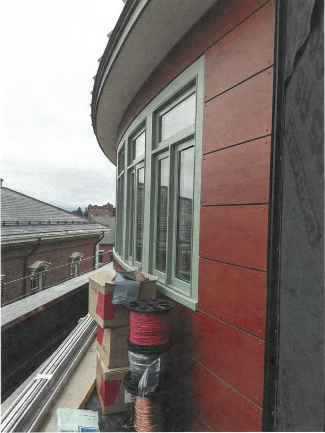
EXPOSED FASTENERS AT 3 PLEASANT ST
