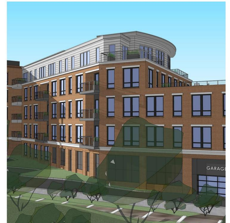
STRONG HORIZONTAL PRECAST BAND CAPS OFF THE FIRST FLOOR. A SUBORDINATE BAND SEPARATES THE TOP FLOOR AND THE NEW PRECAST LINTELS SOFTEN THE FACADE. SYMMETRICAL WINDOW PATTERNS WITH SINGLE AND DOUBLE OPENINGS HAVE A DECIDEDLY RESIDENTIAL FEEL
