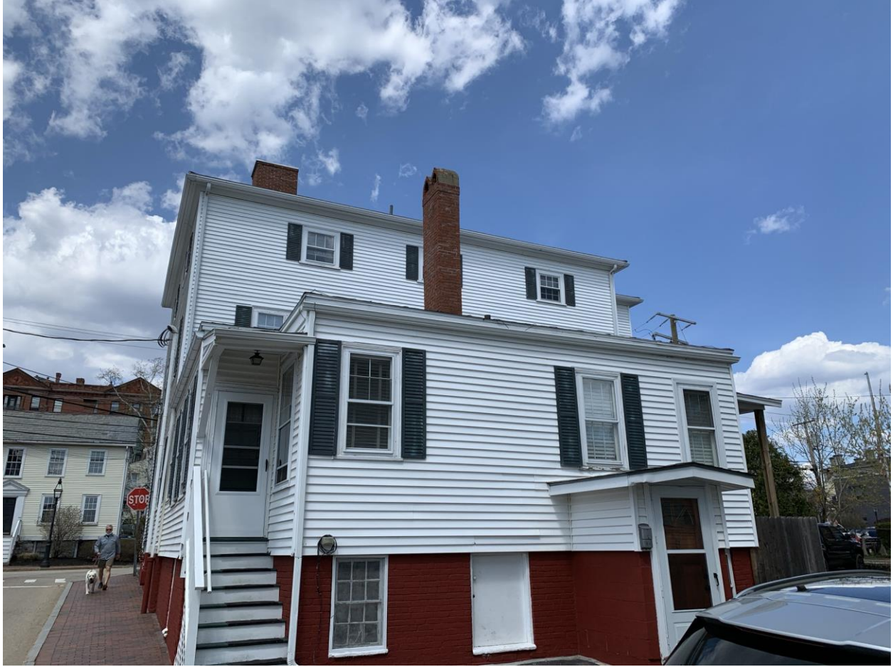
Chimney to be removed on the lower roof at the rear of the building.
