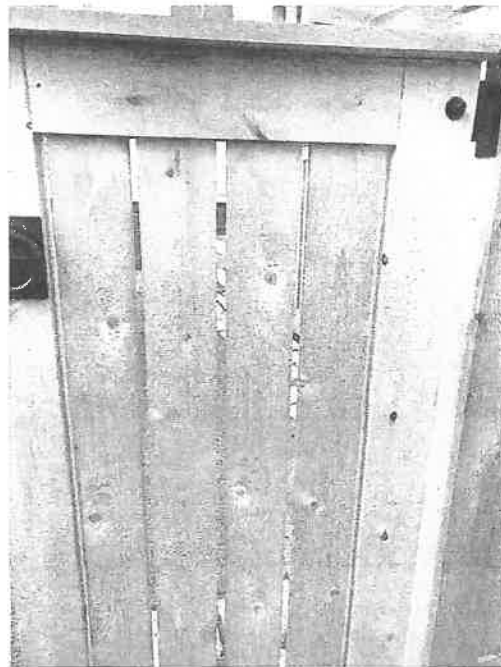
This style with 1/2" narrow gaps would be placed on the side of the cooling unit facing the street
