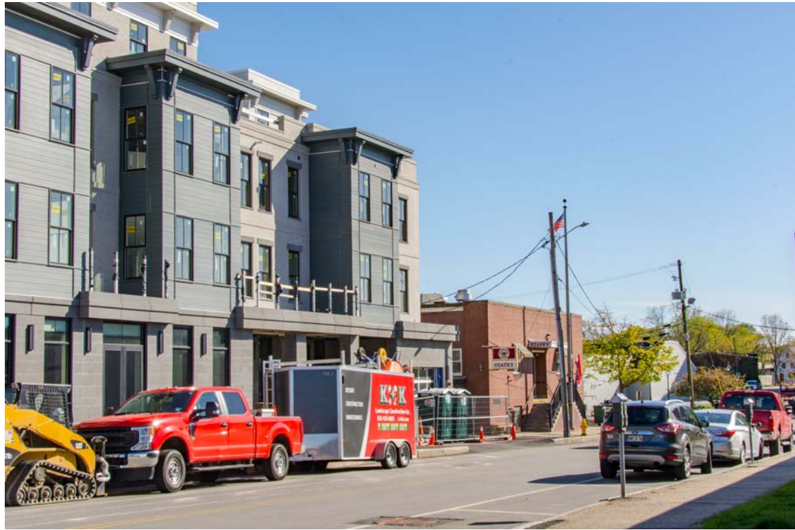
EXISTING PICTURE FROM DEER STREET AND MAPLEWOOD AVE INTERSECTION
