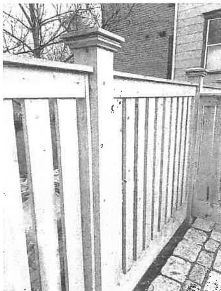
This style with 2" gaps would be in front of the cooling unit facing Side (neighbor) where the fan needs Ventilation.
