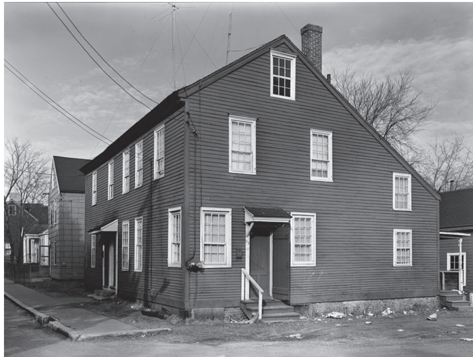
4 SOUTH EAST FACADE
