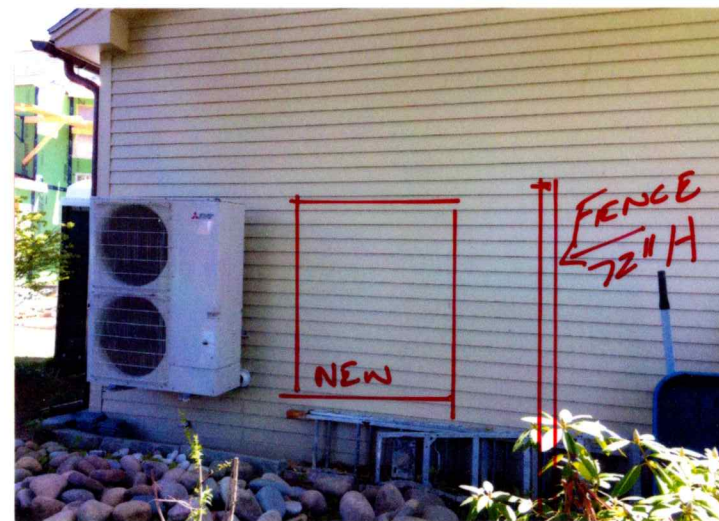
HEAT PUMP LOCATION
