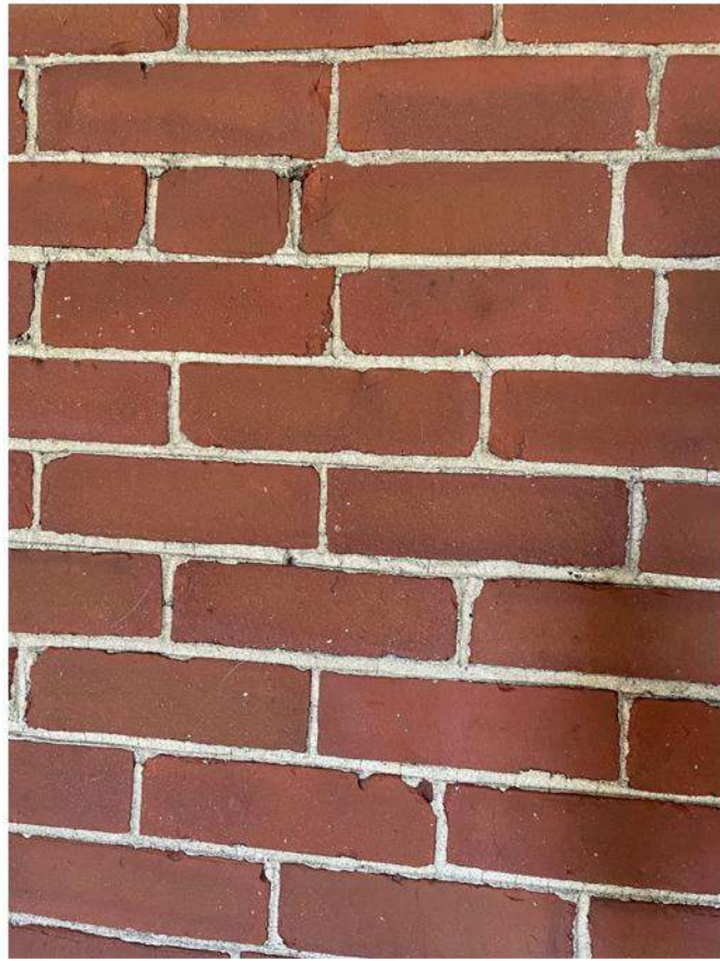
1. Existing Brick Finish (cleaned)
