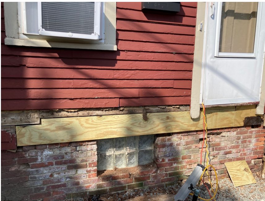
Exhibit 3: Replacing sheathing with \frac{3}{4} " PT plywood
