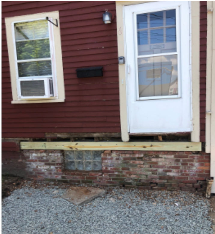
Exhibit 3: Replacing sheathing with \frac{3}{4} " PT plywood
