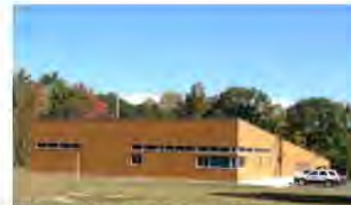
Madbury Water Treatment Facility on Freshet Road
