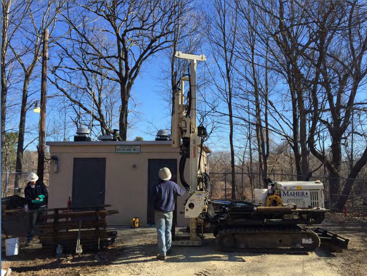
Greenland Well Replacement
