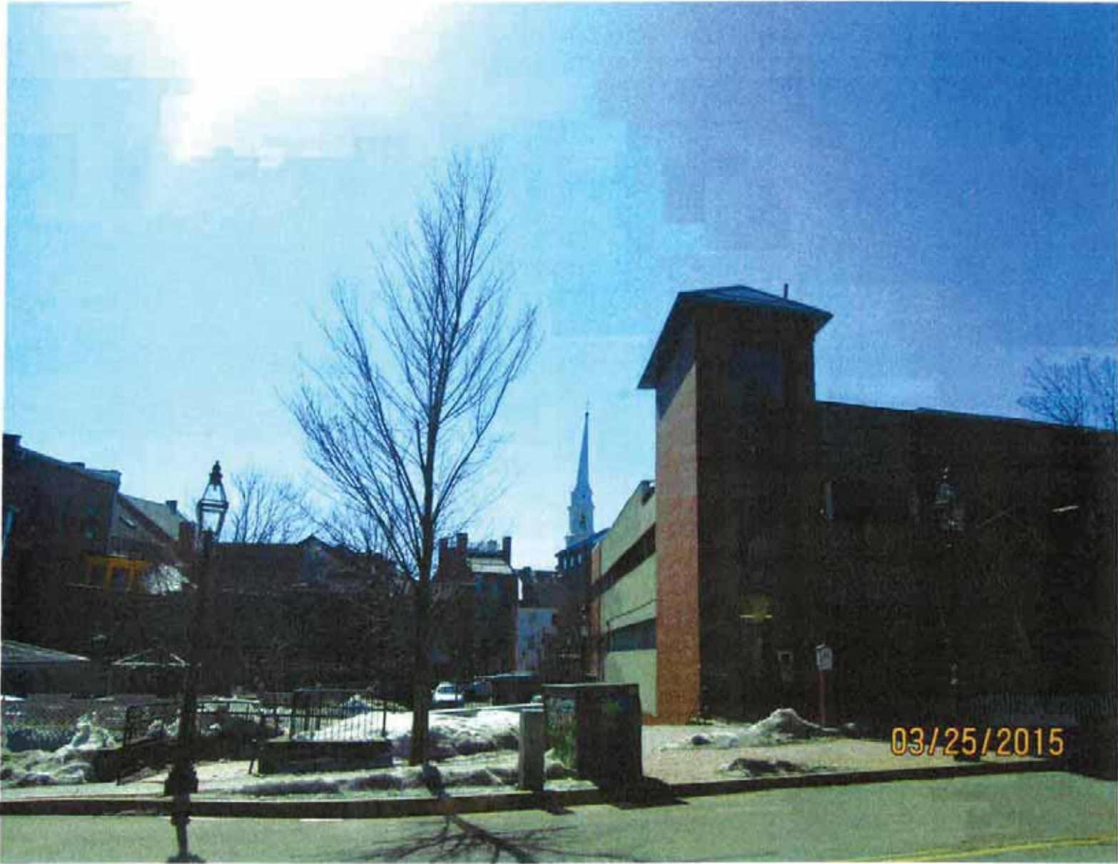
Alley to Ladd Street after
