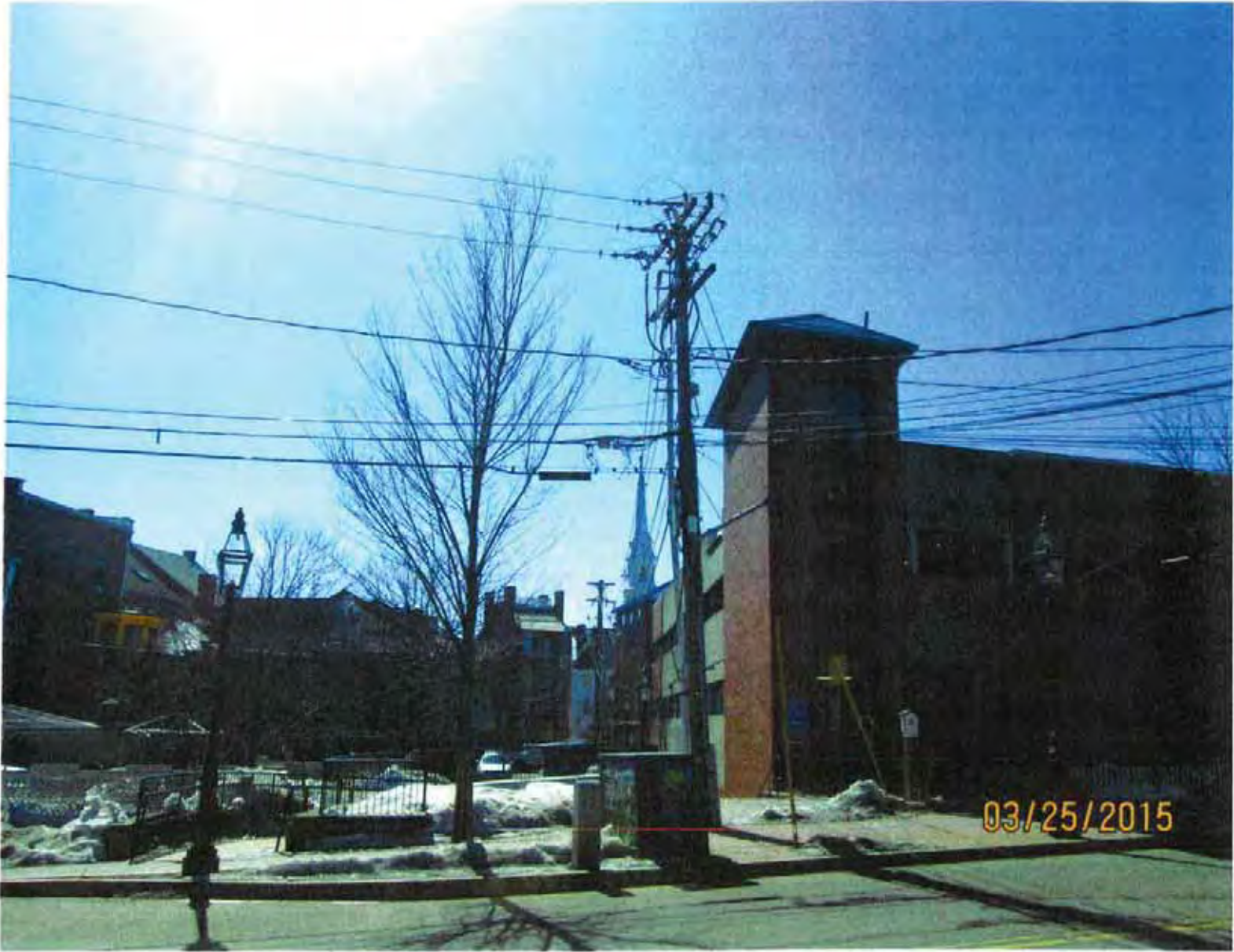
Alley to Ladd Street before
