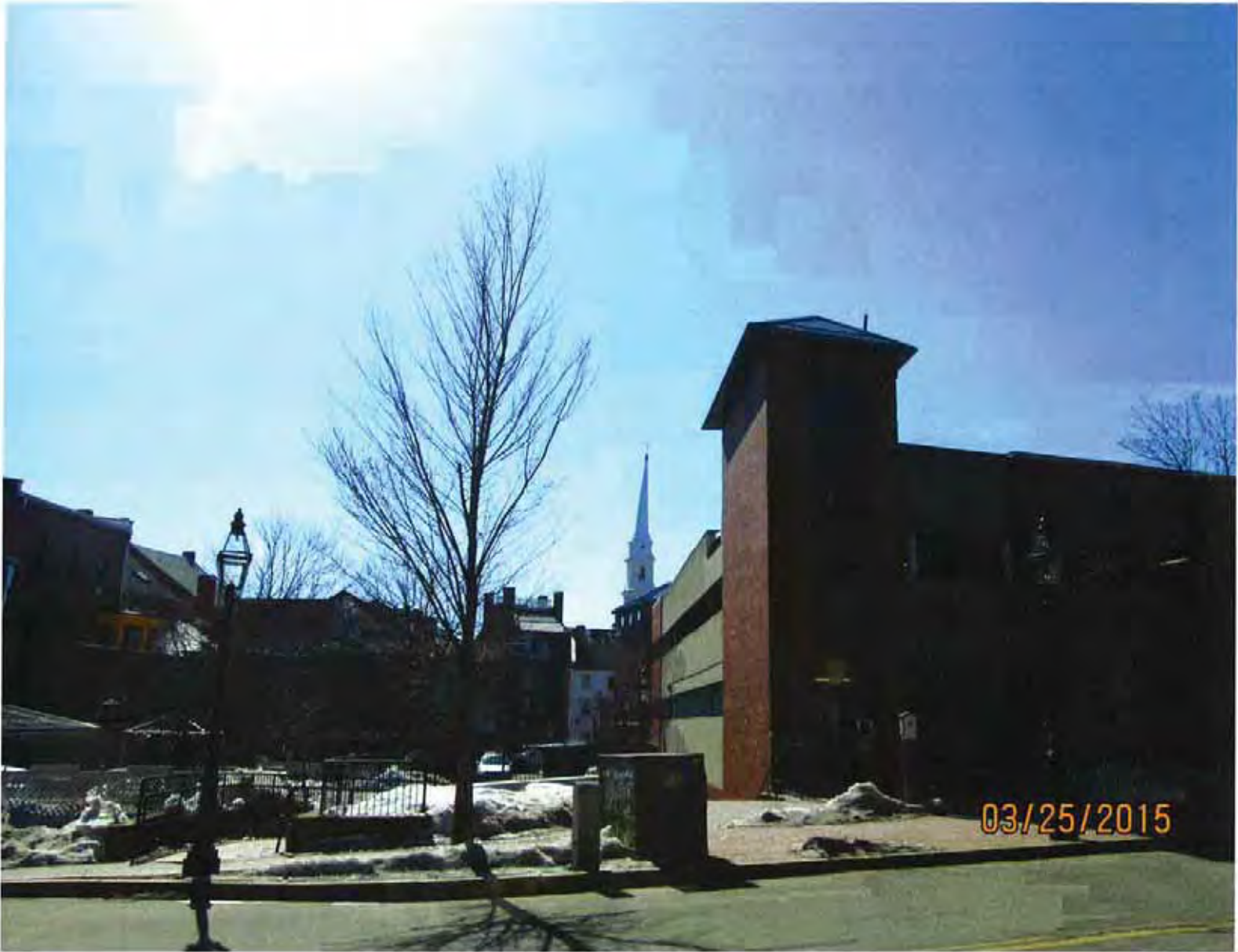
Alley to Ladd Street after
