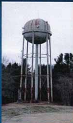
Existing 400,000 Gallon Water Tank
