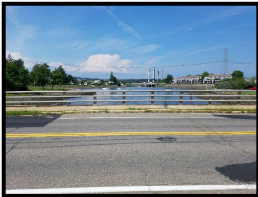
Typical Pavement Condition
