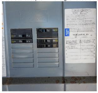
The Hanover St Signal cabinet subpanel is fed from the Deer St cabinet with a 60 Amp double pole breaker. Install a new Square D QO breaker for the lighting in the sub-panel. Pass through the cabinet wall with the wire and into the conduit system which begins inside the cabinet. The 20 amp breaker shown below is the only breaker currently in the panel and runs the signal. Picture of inside the Hanover sub-panel:
