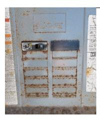
The new Congress St Signal cabinet has no panel or subpanel. Provide new "din rail" style breaker in the empty space inside the cabinet and label it properly to maintain UL rating.
