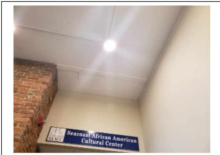
4. Suspect textured surfacing present on the high ceiling in front of the public restrooms.
