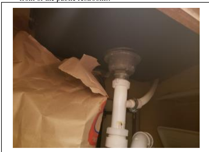
6. ACBM sink basin undercoating located in the Kitchenette.
