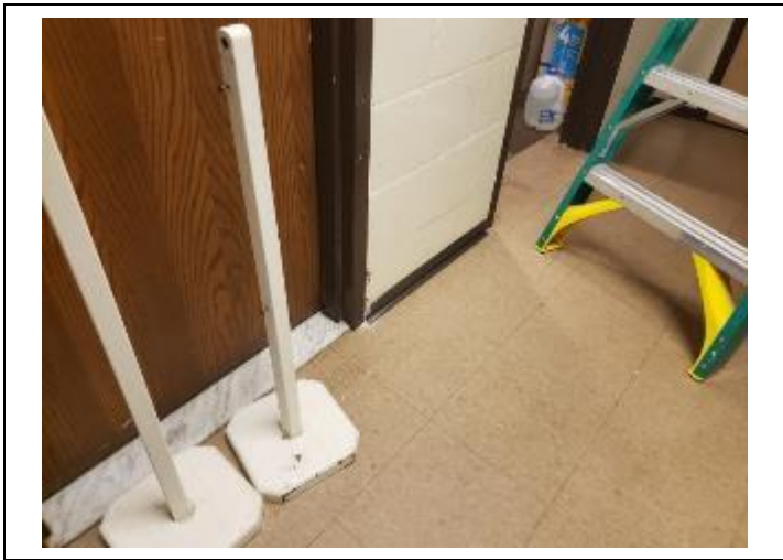
7. ACBM 12" tan floor tile with ACBM black mastic in the hallway outside the staff restrooms.
