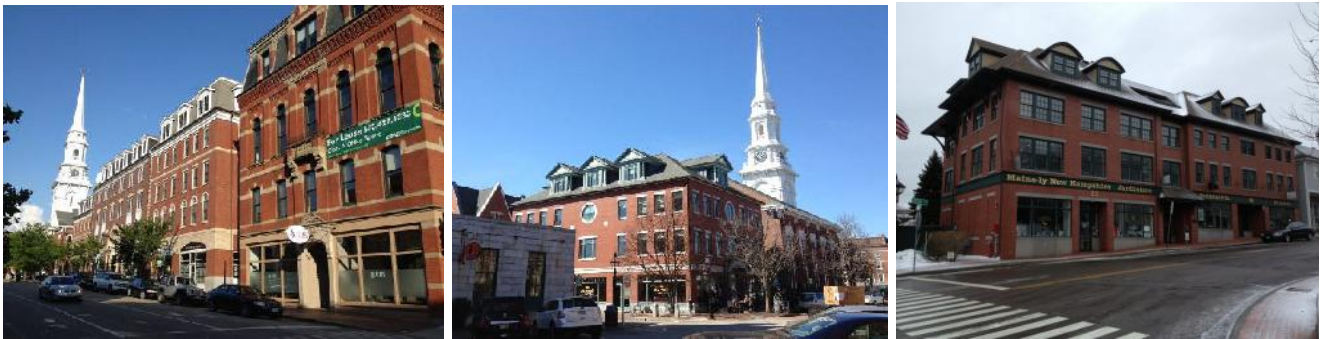
Figure 4 – Examples Large Buildings in the early 21 st Century with a Low-Differentiated Design
