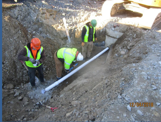
Yard Piping & Utilities
