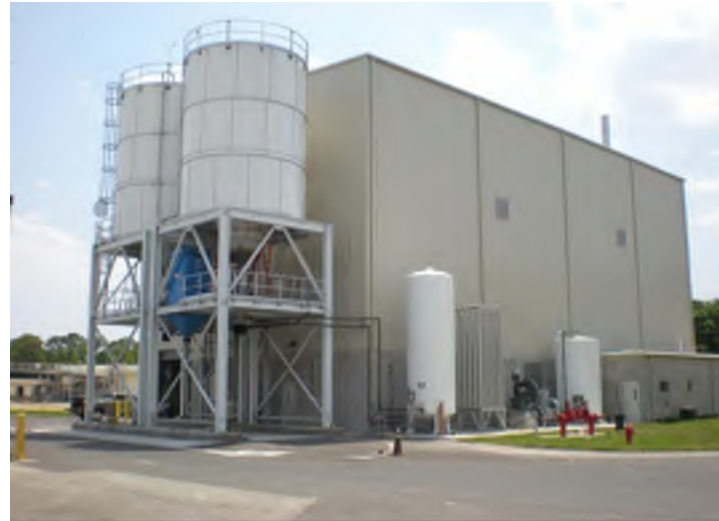
Regional Drying Plant Manatee County, Bradenton, FL
