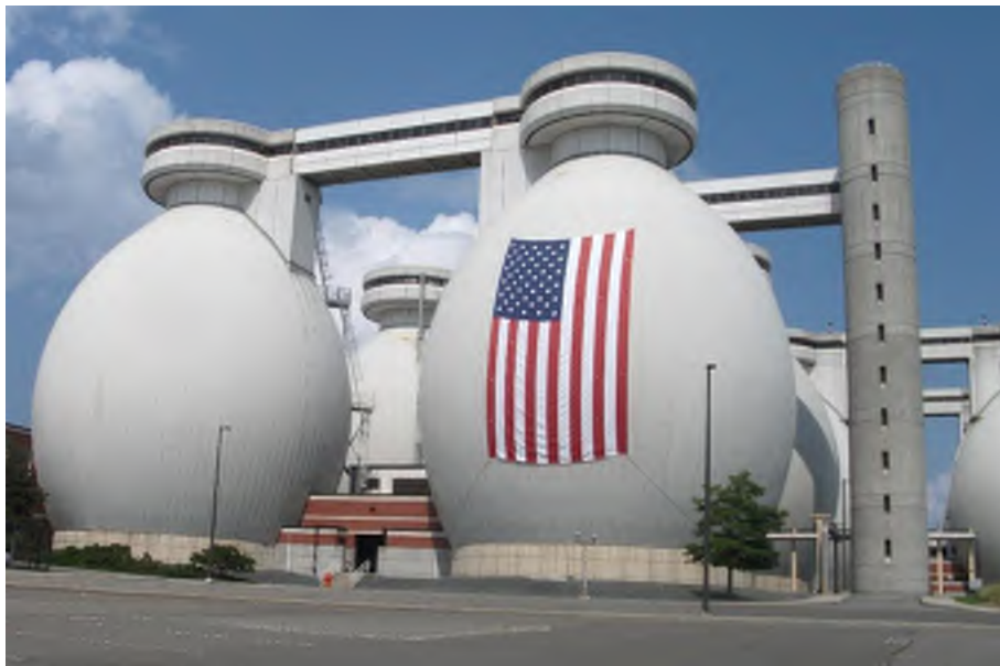
Figure 2-6. Egg-shaped digesters at the Deer Island Treatment Plant, Boston, MA
