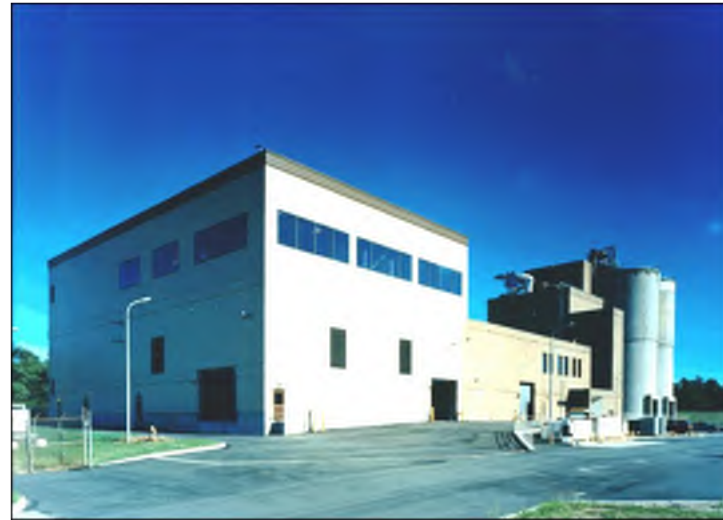
Integrated dewatering and drying, Ocean County, NJ
