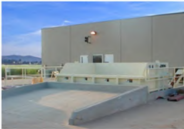
Figure 2-3. Trucked cake receiving stations Courtesy of Schwing Bioaset and Putzmeister
