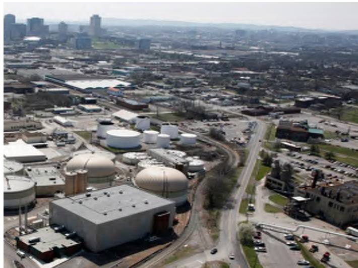
Integrated dewatering and drying, Nashville, Tennessee
