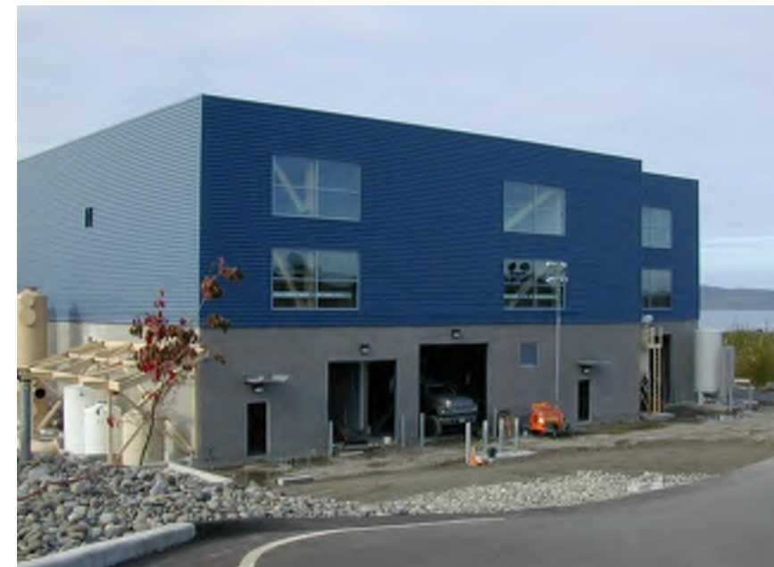
DDS 20 located Pierce County, WA – In service since 2004
