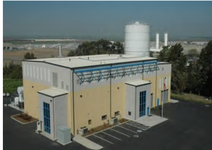
Integrated dewatering and drying facility, Sacramento, CA
