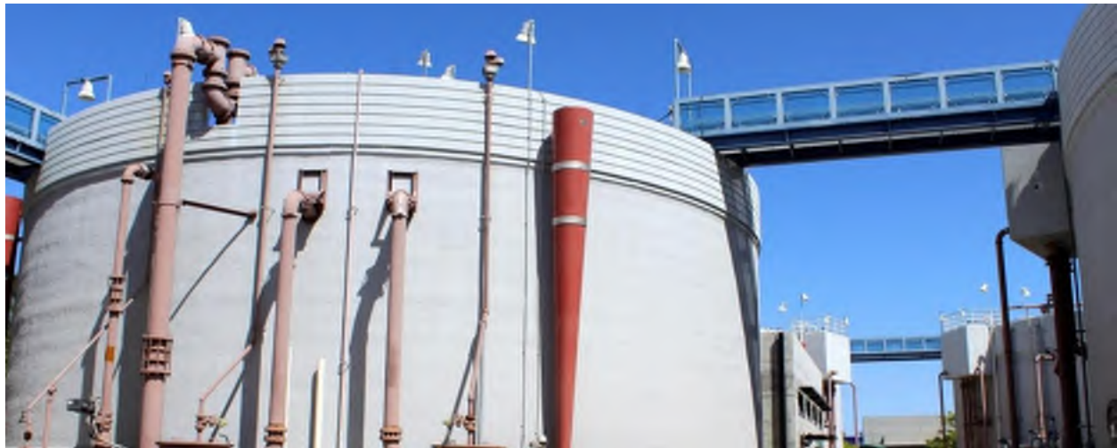
Figure 2-5. Conventional mesophilic digester at the City of San Diego, California
