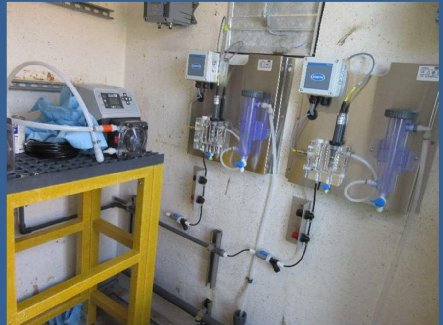
Chlorine Contact Tanks
