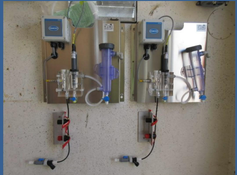
Chlorine Contact Tanks
