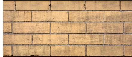
Yellow Brick - A hard, dense, fired-clay, regularly shaped building component made from high lime content clay.
