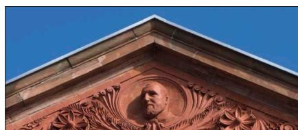
Terra Cotta - A fired-clay, non-structural building component; used for ornate details.
