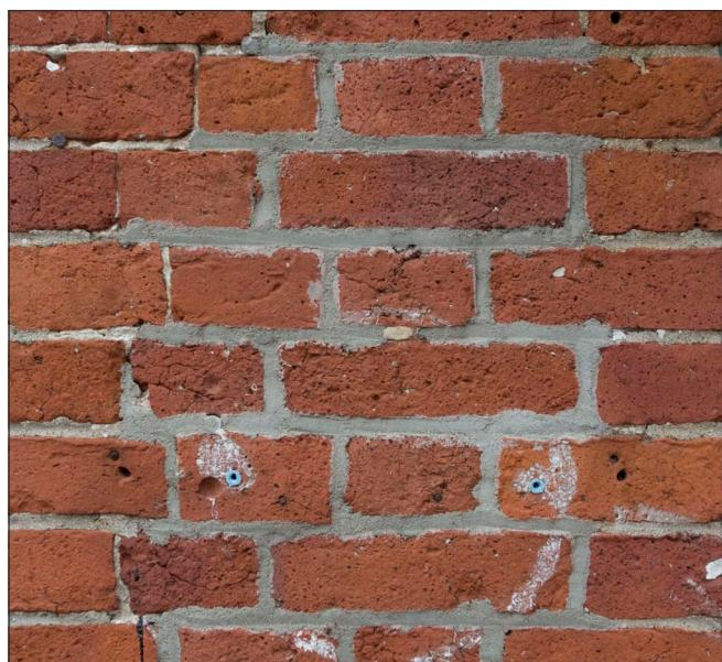
*The central bricks have been repointed with what appears to be a Portland cement mortar that is harder than the hand made brick. In addition, the mortar color and tooling is a poor match for the original mortar.*
