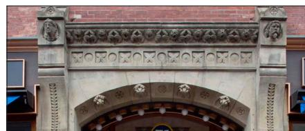
Limestone - A sedimentary rock; used for walls, window sills and lintels and trim.
