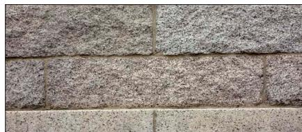
Granite - A hard rock consisting of a small, yet visible, grains of minerals; can be highly polished or textured.
