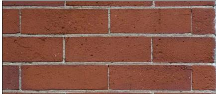
20th Century Brick - A hard, dense, fired-clay, regularly shaped building component; sometimes with a glazed surface.
