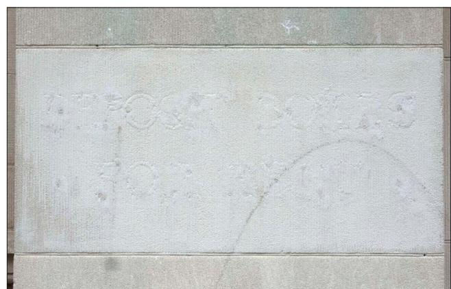
*It appears that an aggressive treatment was used to clean the limestone surface, resulting in a “bleached” effect when compared to adjacent stones. Although it is preferable to clean and entire wall surface, if spot cleaning is being considered, it is preferable to clean entire stone units ending at mortar joints as shown.*
