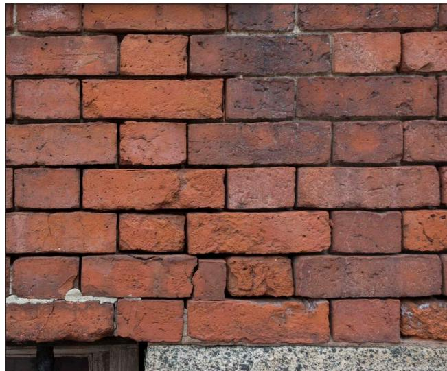
*The mortar has weathered from most of the brick joints, reducing the structural capacity of the wall. The surface of some bricks has spalled, and a settlement crack has developed near the corner of the window.*
