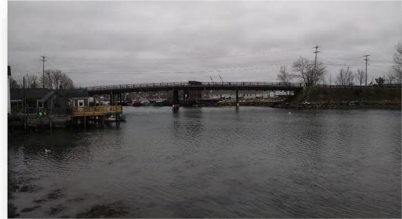
**Description:** A recently completed bridge inspection found the Peirce Island Bridge needs to be replaced within the next 5 to 10 years. Interim repairs have been completed to ensure use until 80% State DOT bridge funds are available. Replacement of the bridge will start after the Peirce Island Wastewater Treatment Facility Upgrade project is completed.
