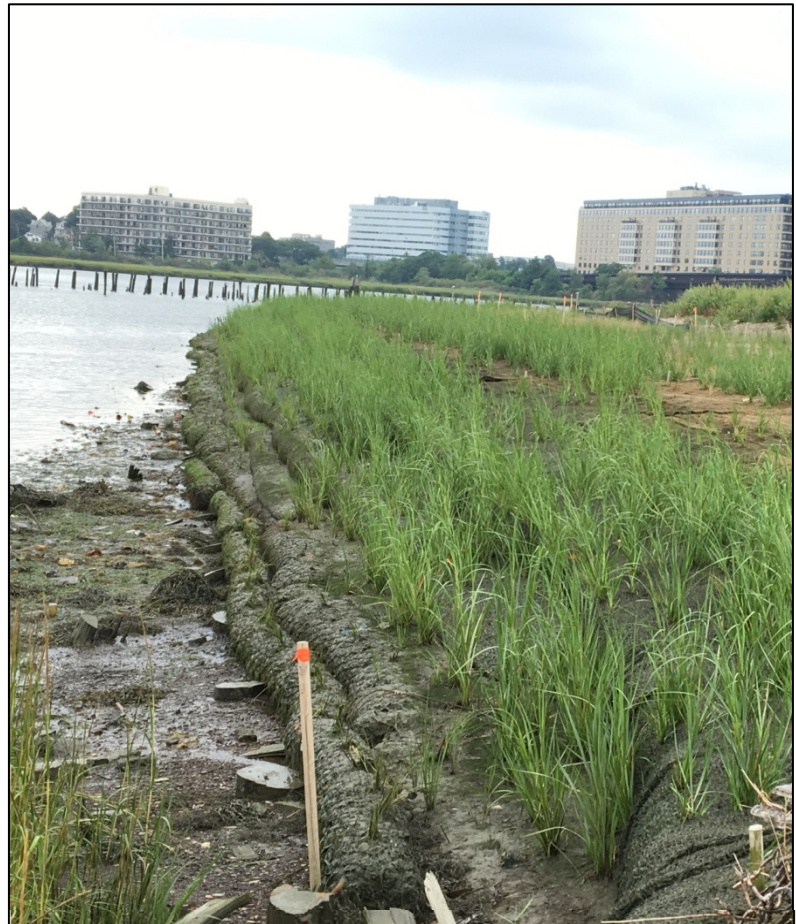
View of coir log installation on Neponset River held fast with Duck Bill Anchors. Photo taken after two growing seasons. Spartina alterniflora well established.
