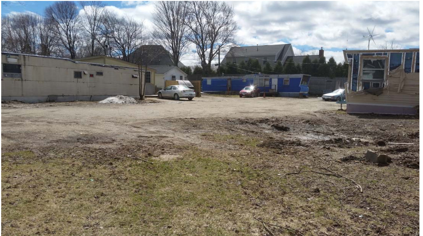
Photo looking southwest out at the existing park and gravel parking area from the rear the of the cottage (to be demolished) and the rear of the garage/apt. (to be demolished).
