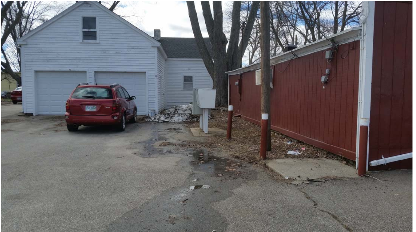
Photo looking west at the side of the red former store building (to be demolished), the front of the white garage/apartment building (to be demolished) and the mailbox (to be relocated).
