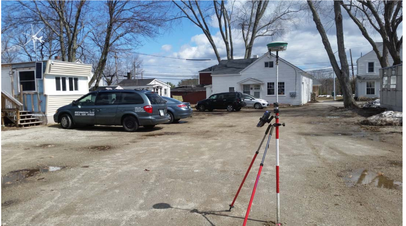
Photo looking east at the rear of the cottage (to be demolished) and the rear of the garage/apt. (to be demolished).
