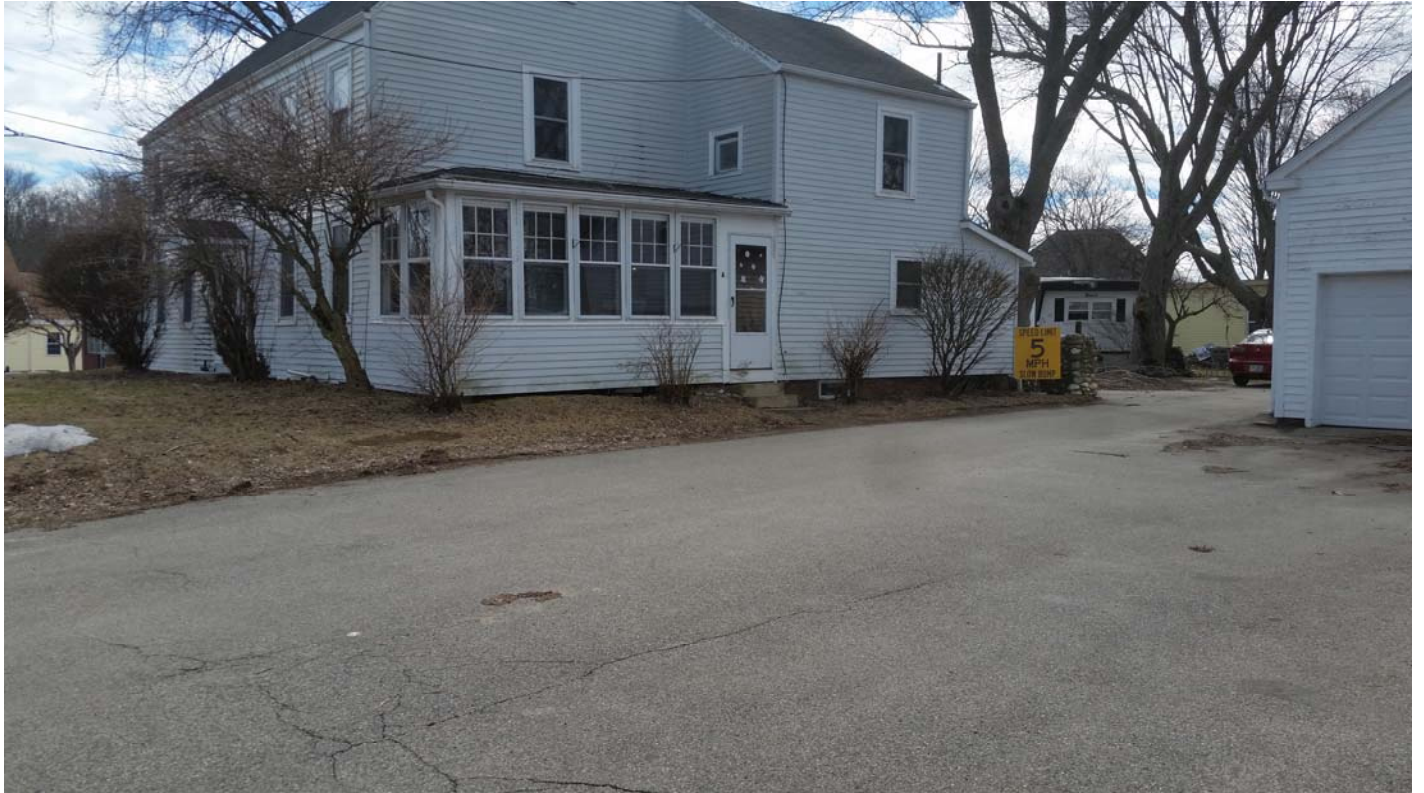
Photo looking south at the side of the 3 unit apartment building and park entrance.
