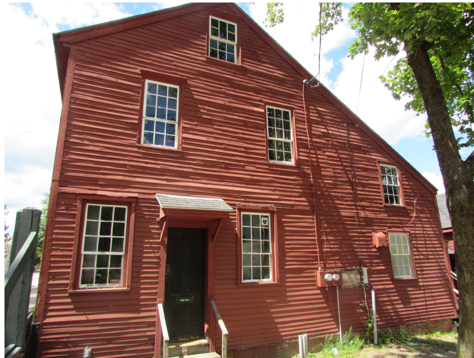
5 SOUTH EAST FACADE
