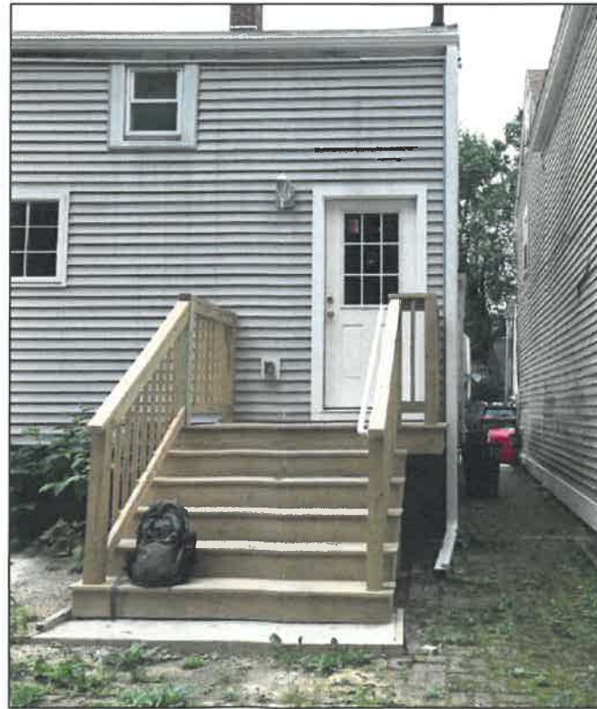
REBUILT EXIT STAIR
