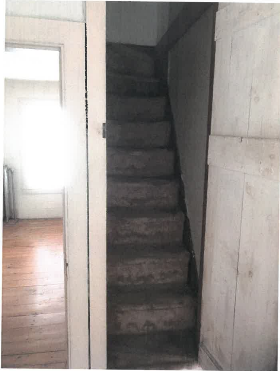
Current stairway to third floor
