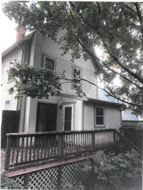
Current First Floor Bathroom/Entry Add-On
