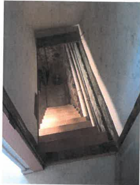
Existing interior stairway to basement
