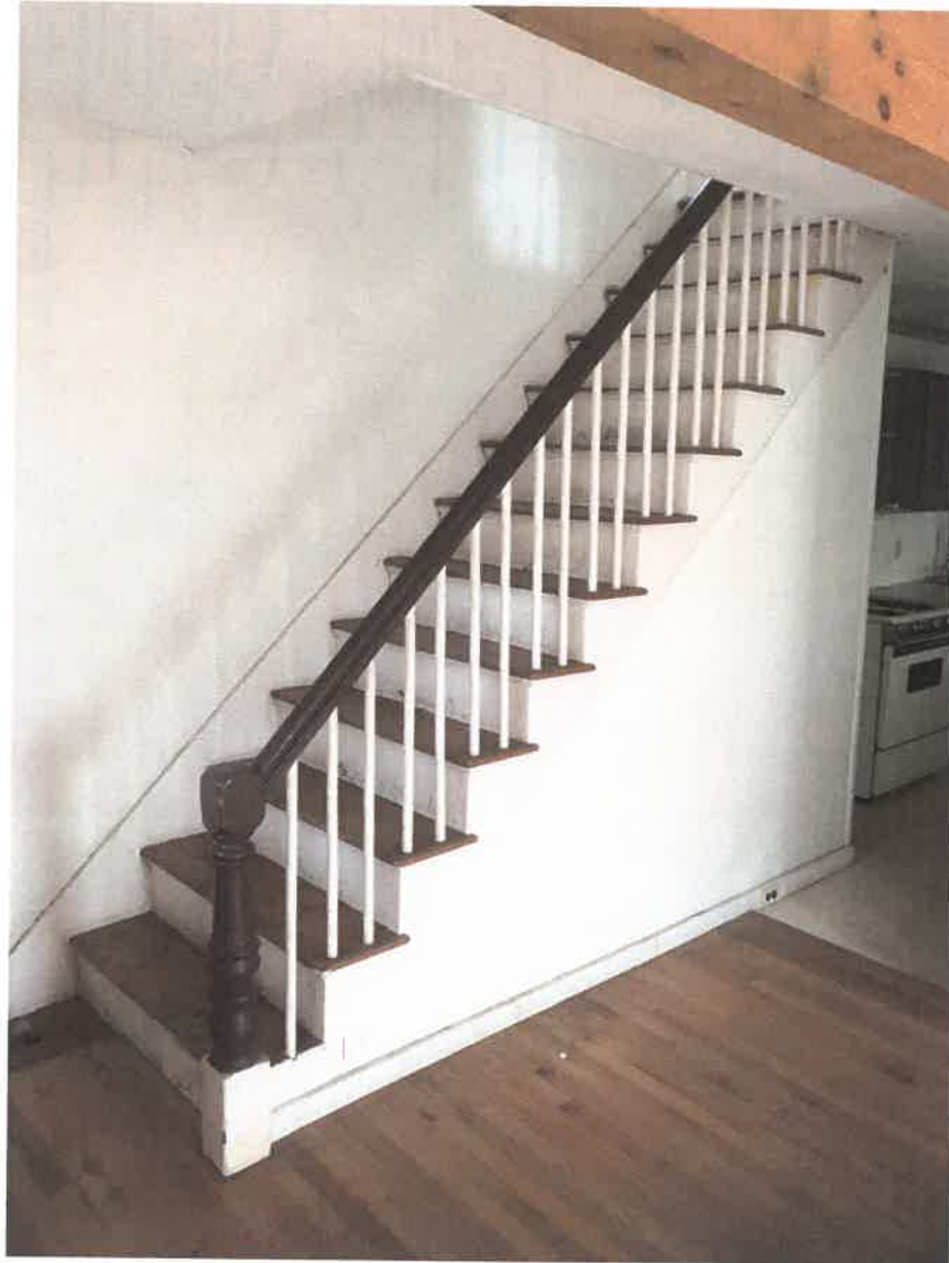
Current stairway from first to second floor
