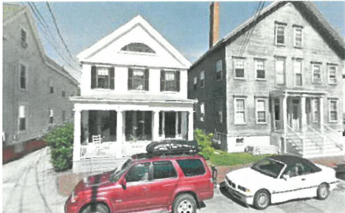
A No visible view of changes from street front
