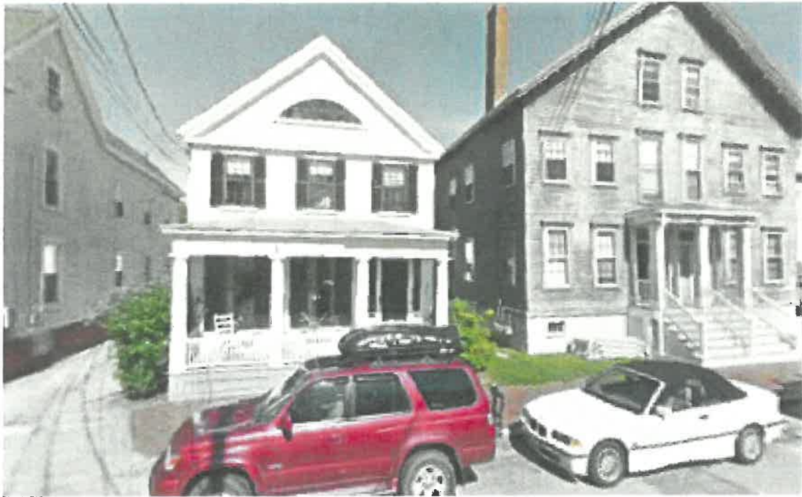
A Existing view from street front
